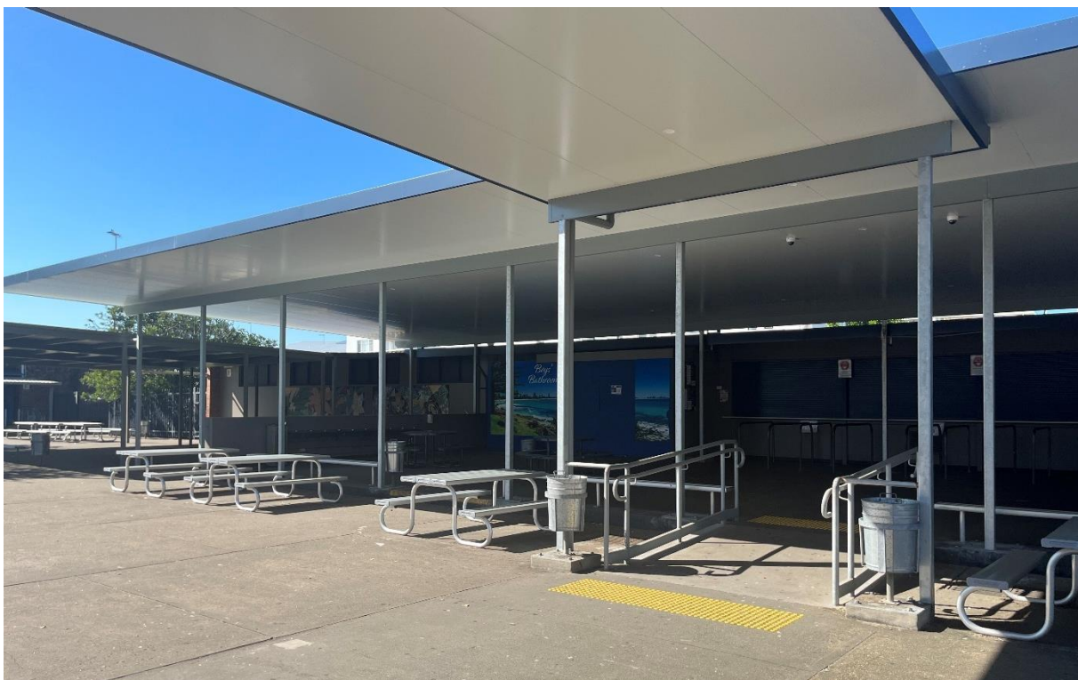
Figure 6: Existing bathrooms and canteen (Building B) proposed to be demolished, viewed from central quadrangle
