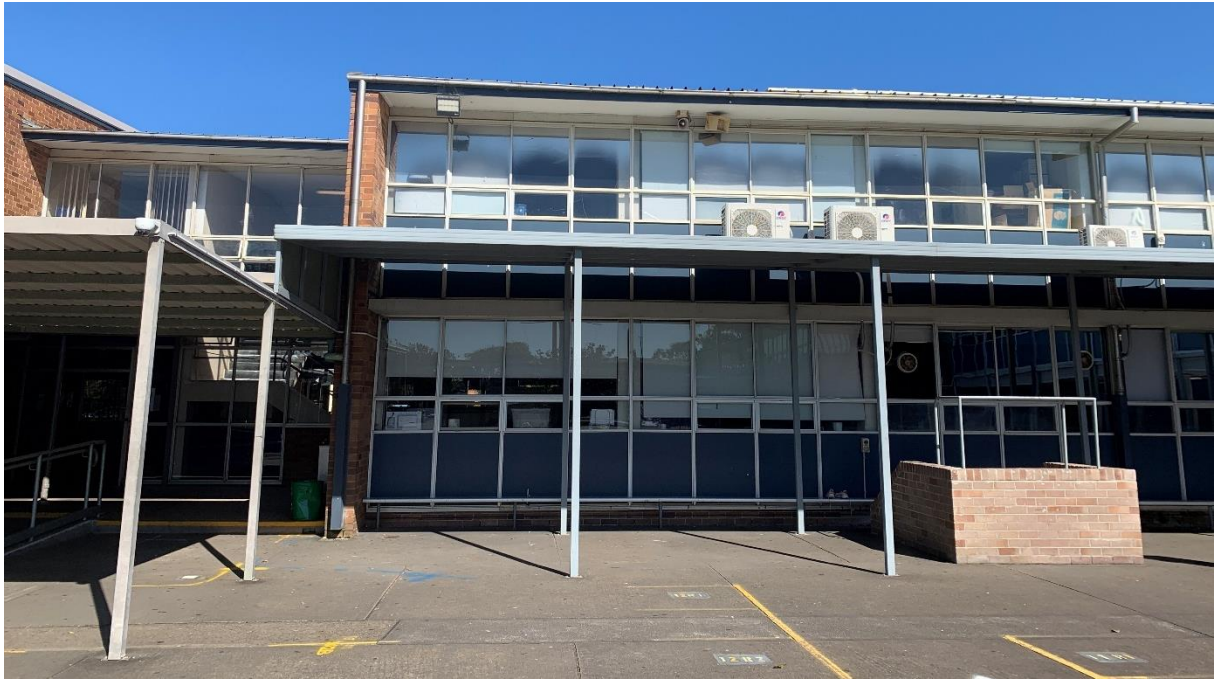
Figure 9: Existing administration building (Building D), viewed to south west from central quadrangle
