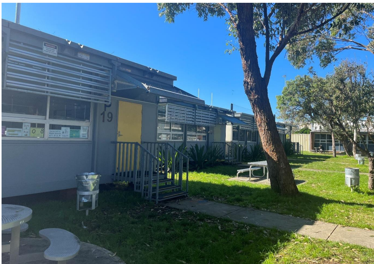
Figure 13: Existing demountable classrooms, viewed to north east
