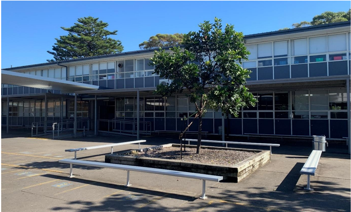
Figure 11: Existing Building E, viewed from central quadrangle
