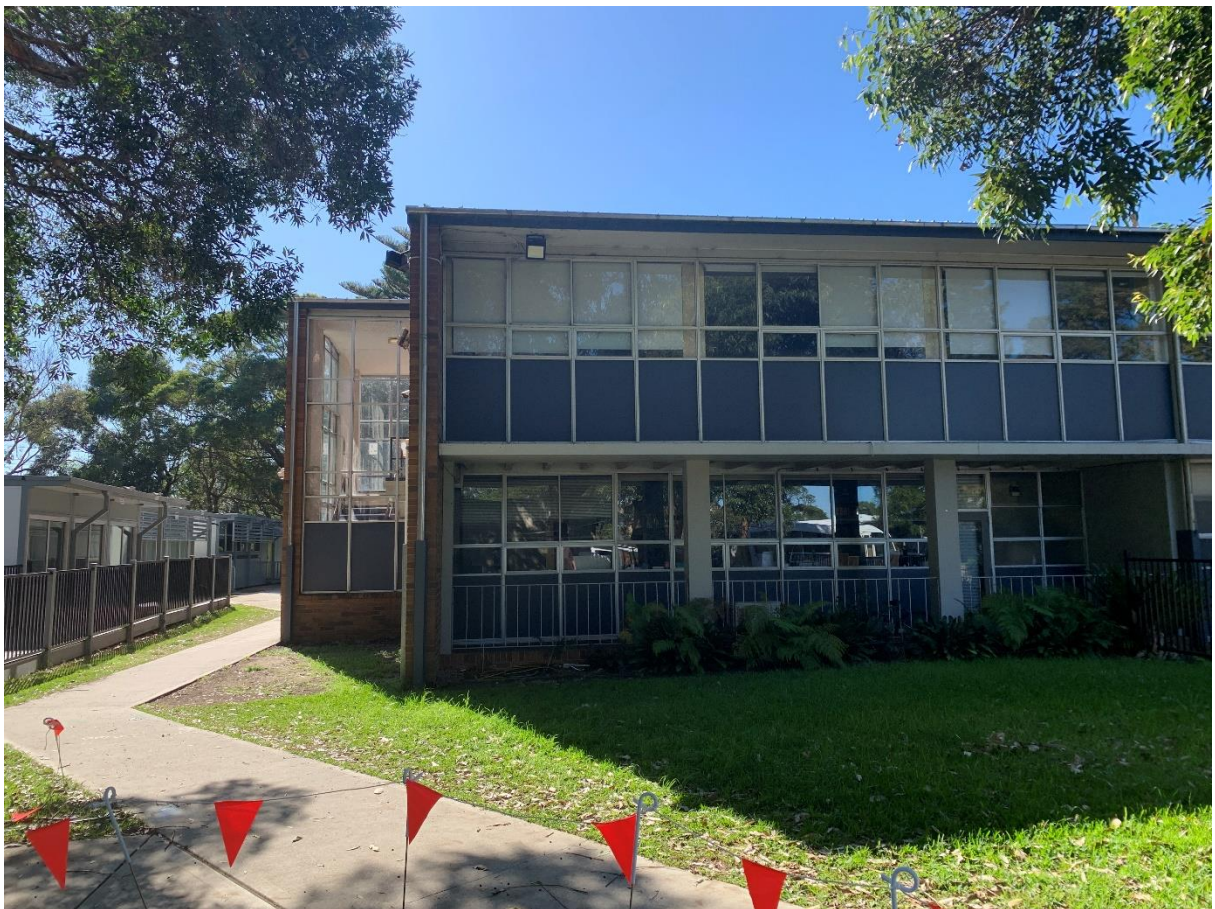
Figure 10: Existing administration building (Building D), viewed to south east
