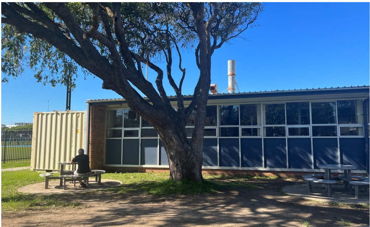
Figure 8: Existing tech rooms (Building C) and outdoor seating area, viewed to south east
