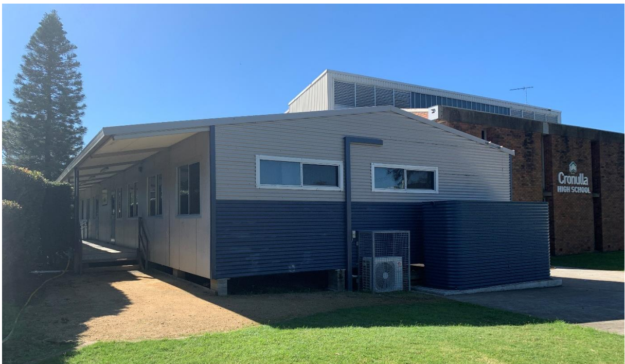
Figure 12: Existing Building I, viewed to north east
