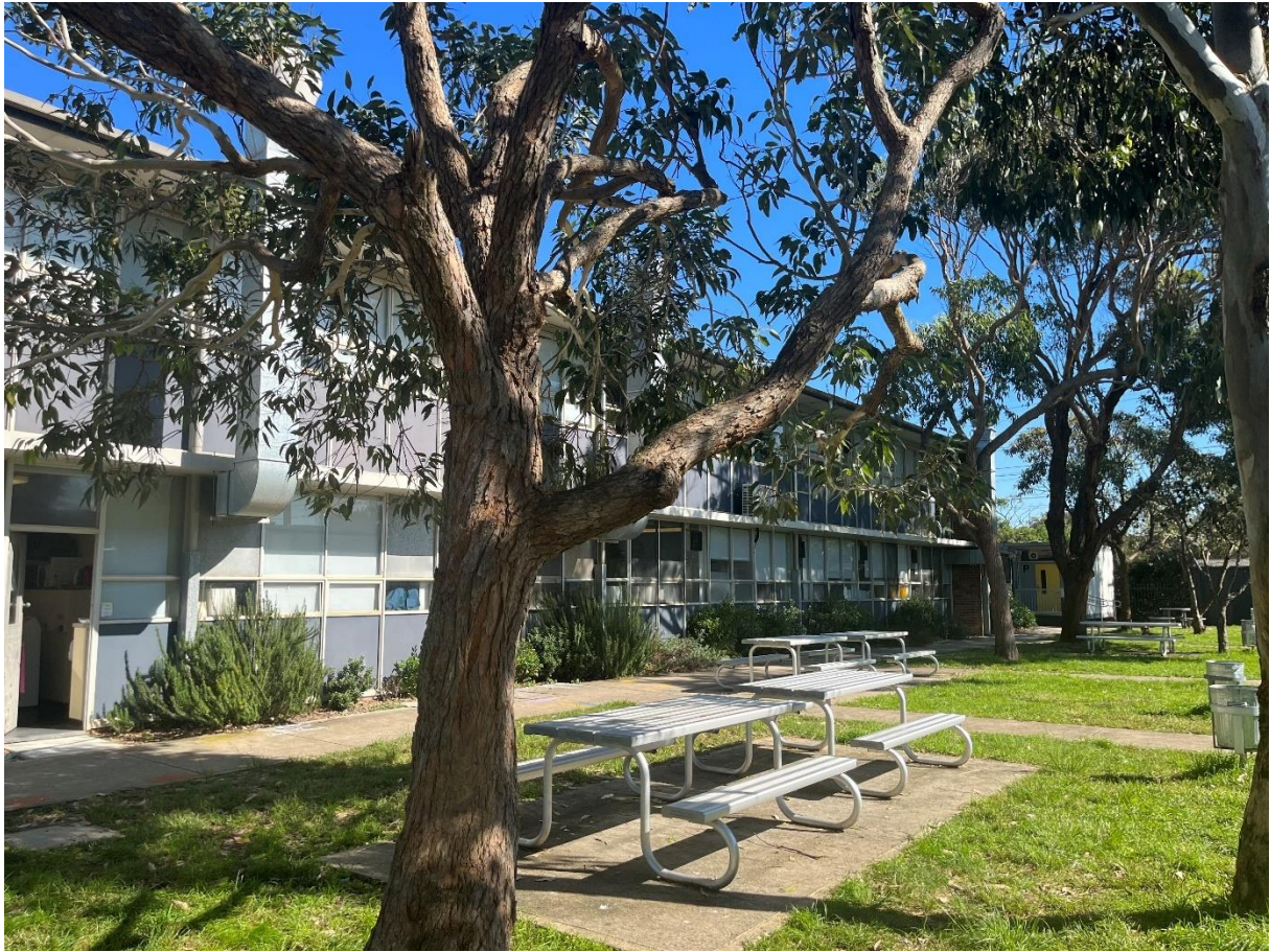
Figure 7: Existing science labs (Building A) and outdoor seating area, viewed to north west
