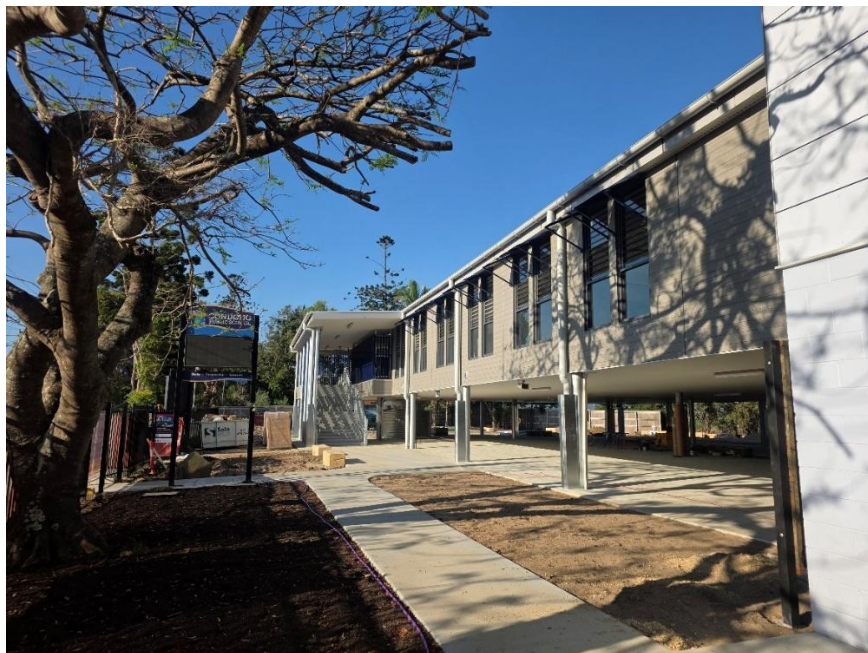
Front of the school ready for new gardens
