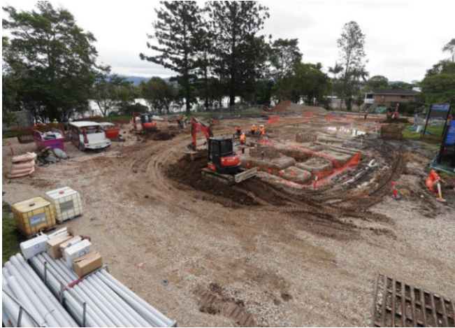
Installing the screw pyles to support the school
