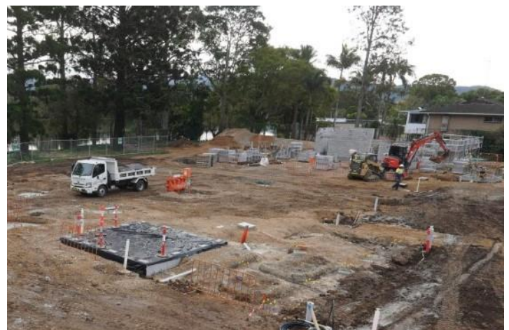
Starting the blockwork on the amenities block
