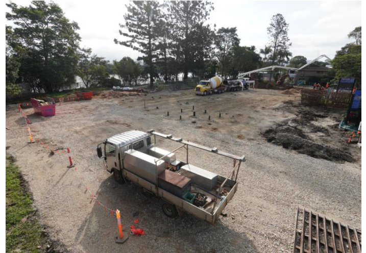
Screw piles all neatly in the ground and capped
