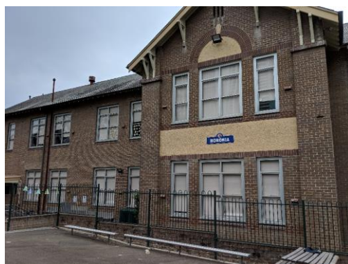
'Building B' Heritage Item
