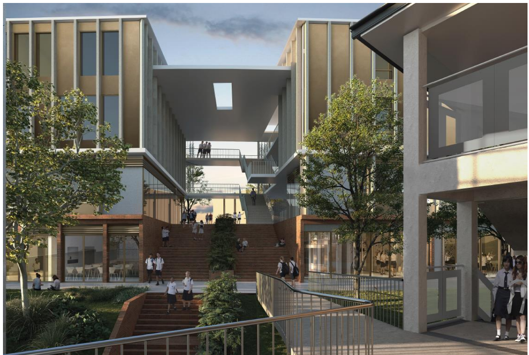
Figure 48 Western façade of Building Q indicating the void in between the two structures
