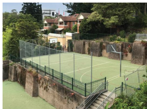
'The Lowers' – Retaining Wall Heritage Item
