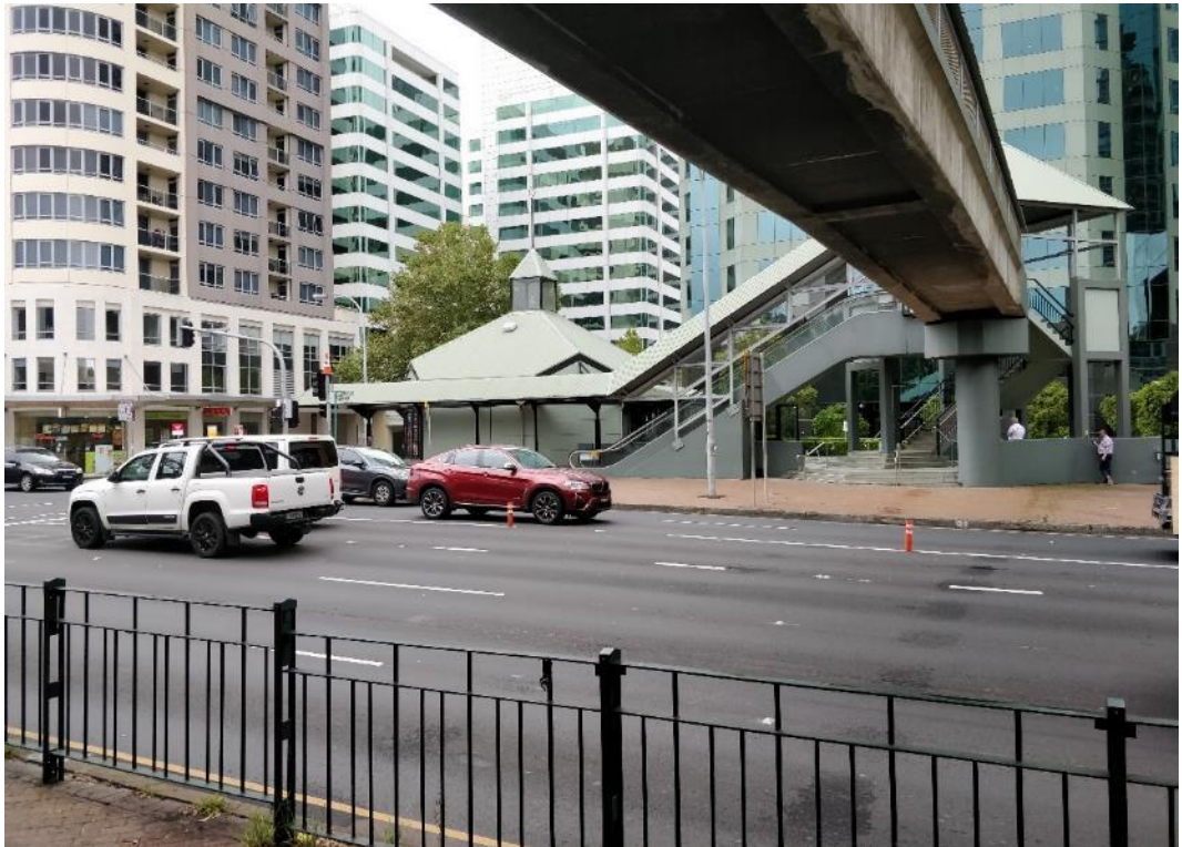
Figure 10 Pedestrian overpass on Pacific Highway near entry to Chatswood Public School
