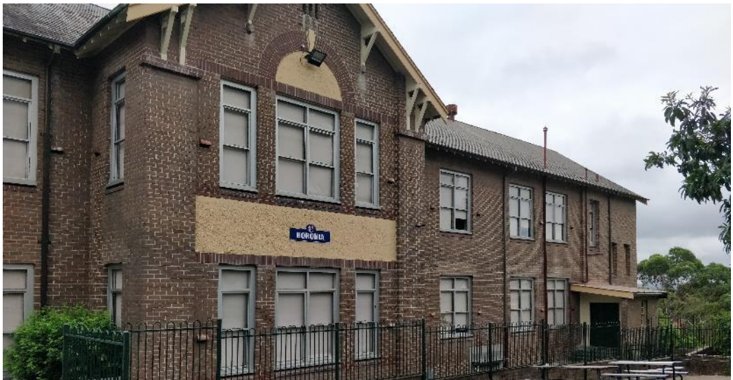
Figure 51 Building B façade (part two-storey, part four-storey)
