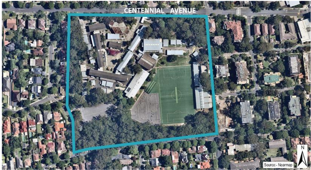
Figure 7 Aerial photograph of Chatswood High School site
