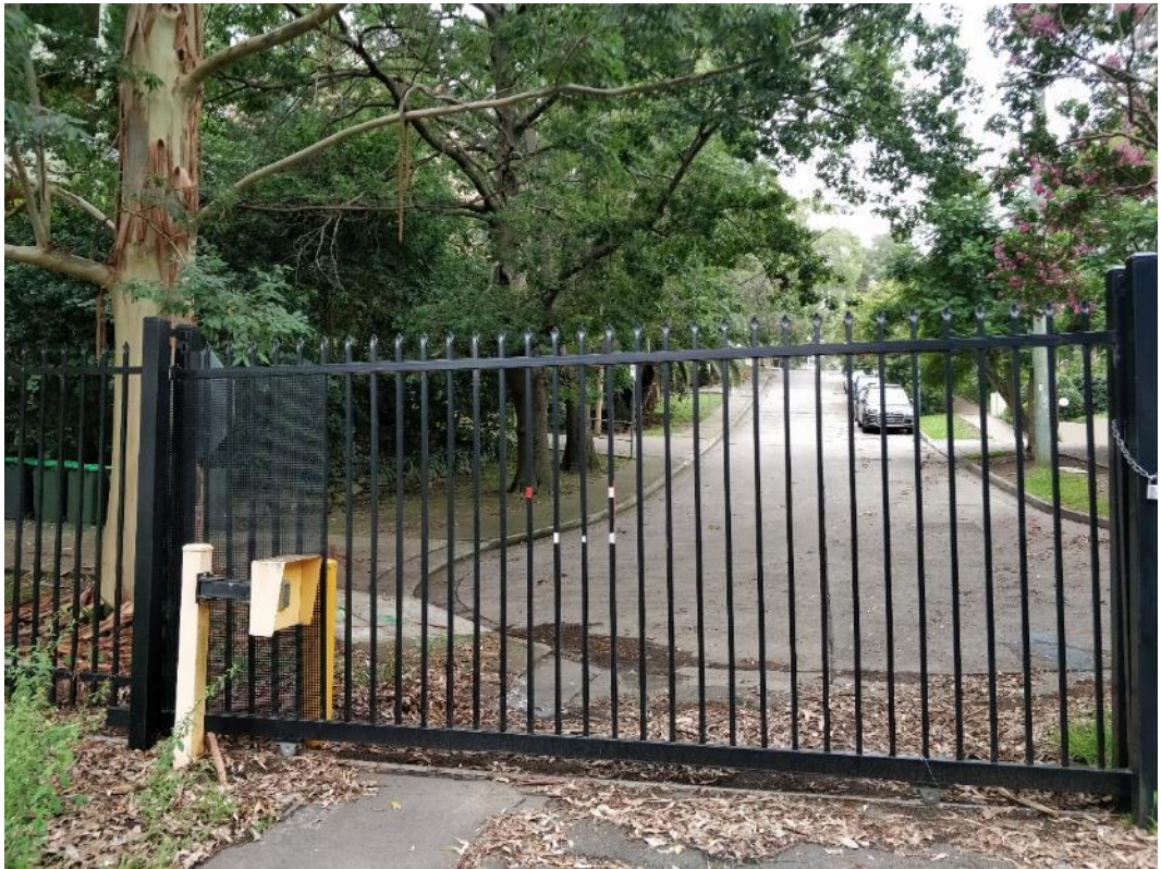
Figure 14 View of vehicular access gate at end of cul-de-sac on Oliver Road
