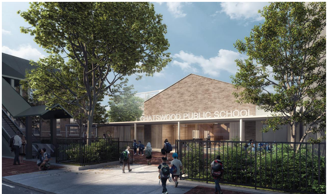
Figure 37 Perspective of Building G from Pacific Highway with Building P2 in the background.
