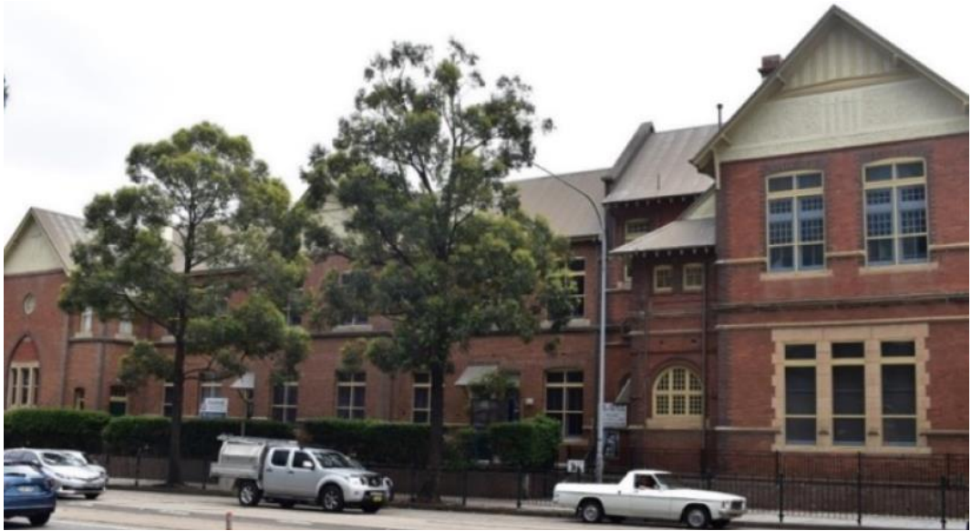
Figure 50 Façade of Building A
