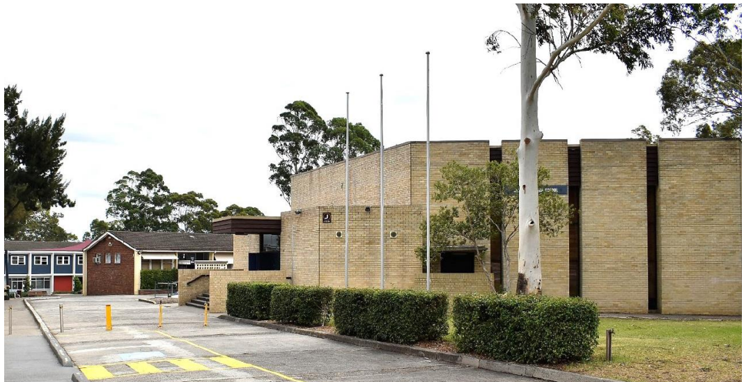
Figure 3 Chatswood High School (Building J) from Centennial Avenue
