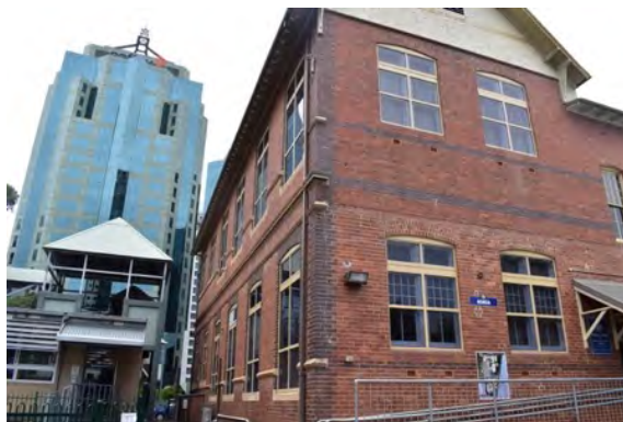
Figure 17 Photograph taken from the north western side of Building A showing the western façade of Building A with 1902/03 and 1915 phases of development as evidenced in the change of brick colour. Source: May Willard 11 th January 2018.
