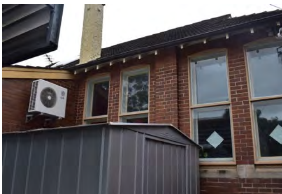
Figure 20 Photograph taken from directly in front of the 1908 extension, with sandstone copings to windowsills and rough cast chimney. Source: May Willard 11 th January 2018.
