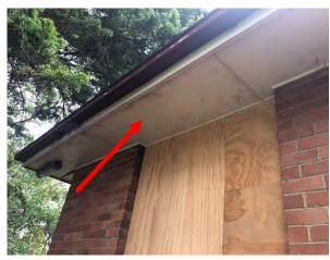
Photo 36: Building C, asbestos containing fibre cement eaves
