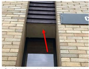
Photo 54: Building J, suspected asbestos containing fibre cement sheeting to eaves above windows
