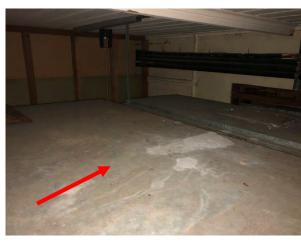
Photo 15: Building A, lead containing dust to air conditioning loft in Room R0031
