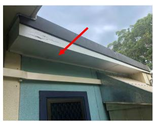
Photo 26: Building D, asbestos containing fibre cement sheeting to the external eaves of Room  $\mbox{R0026}$
