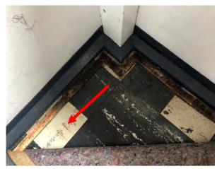
Photo 24: Building D, asbestos containing white vinyl floor tiles to Room
