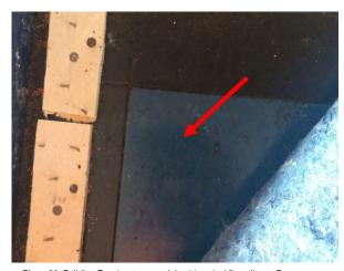
Photo 30: Building E, asbestos containing blue vinyl floor tiles to Room R1001
