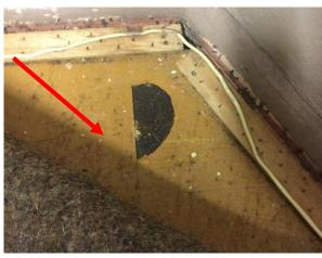
Photo 3: Building A, asbestos containing mustard vinyl floor tiles to Room
