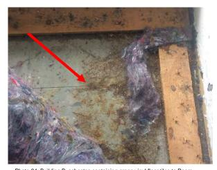
Photo 24: Building B, asbestos containing green vinyl floor tiles to Room  ${\sf R}0003$
