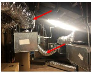
Photo 45: Building H, suspected SMF insulation to air conditioning ducting
