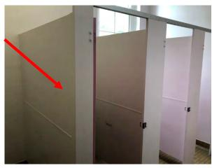
Photo 27: Building B, asbestos containing fibre cement cubicle partitions to Room R0004
