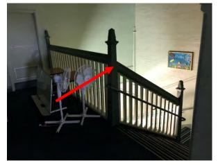
Photo 19: Building A, lead based green paint to stair handrail in Room R1020
