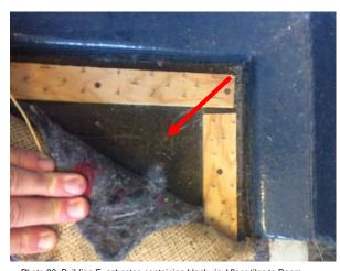
Photo 28: Building E, asbestos containing black vinyl floor tiles to Room R0007
