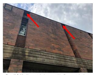
Photo 42: Building H, suspected asbestos containing fibre cement sheeting to eaves above windows
