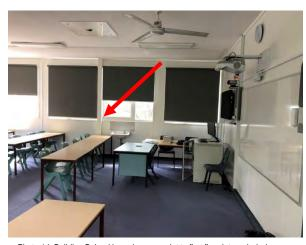
Photo 14: Building B, lead based cream paint to first floor internal windows
