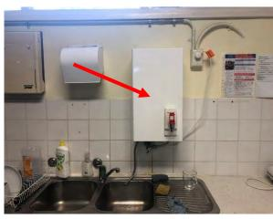
Photo 9: Building A, suspected SMF insulation core to instant hot water system in Room R0014
