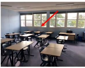
Photo 33: Building E, lead based white paint to Room R1007 windows
