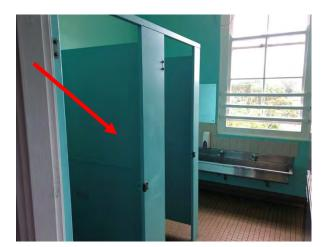
Photo 28: Building B, asbestos containing fibre cement cubicle partitions to Room  $\mathsf{R}1003$
