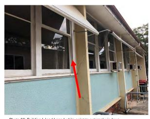
Photo 52: Building I, lead based white paint to external windows
