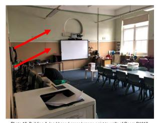
Photo 18: Building A, lead based green/orange paint to walls of Room R1012
