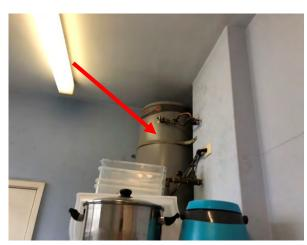
Photo 42: Building H, suspected SMF insulation core to hot water system in Room R0016
