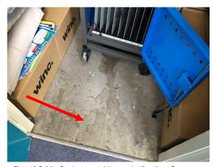
Photo 12: Building B, asbestos containing grey vinyl floor tiles to Room R1004
