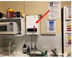
Photo 15: Building B, suspected SMF insulation core to instant hot water system in Room R0007
