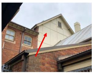
Photo 14: Building A, asbestos containing fibre cement sheeting to south gable
