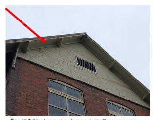
Photo 12: Building A, suspected asbestos containing fibre cement eaves
