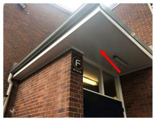
Photo 39: Building F, asbestos containing fibre cement sheeting to east and west entry soffits (R0017 & R0018)
