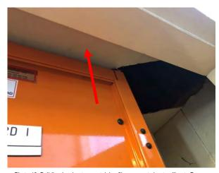
Photo 48: Building I, asbestos containing fibre cement sheet ceiling to Room R0007
