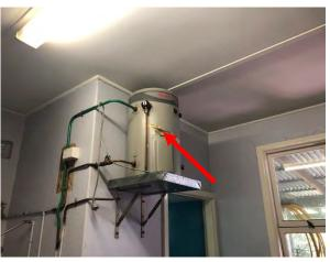
Photo 57: Building AA, suspected SMF insulation core to hot water system in Room R0007  $\,$
