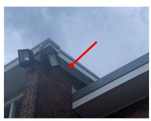
Photo 32: Building E, suspected asbestos containing fibre cement sheeting to eaves
