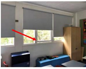
Photo 8: Building A, lead based white paint to Room R1001 windows
