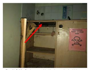
Photo 34: Building C, asbestos containing bituminous pad under sink in Room  ${\tt R0004}$
