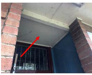
Photo 33: Building C, asbestos containing fibre cement sheeting to Room R0001 ceiling (external soffit)
