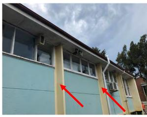
Photo 51: Building I, lead based cream paint to external walls
