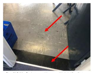
Photo 36: Building F, asbestos containing grey and black vinyl floor tiles to Room R1019
