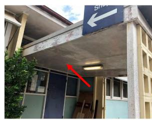
Photo 50: Building I, asbestos containing fibre cement sheeting to external soffit lining (R0017)
