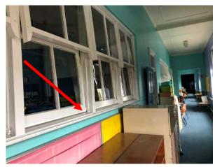
Photo 30: Building B, lead based white paint to windows in Room R1005
