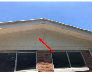
Photo 56: Building AA, asbestos containing fibre cement sheeting to gable panels
