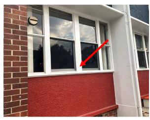
Photo 20: Building C, lead based white paint to external windows
