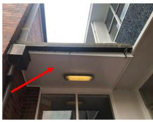
Photo 3: Building A, asbestos containing fibre cement sheeting to east and west entry soffits (R011 & R017)
