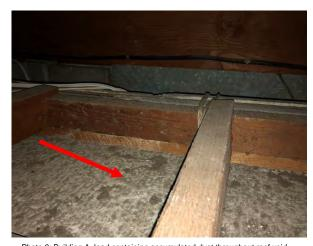
Photo 6: Building A, lead containing accumulated dust throughout roof void
