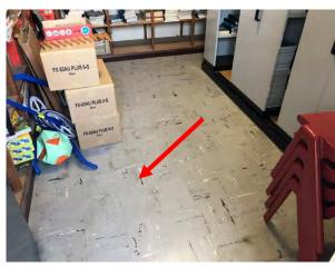
Photo 27: Building E, asbestos containing grey vinyl floor tiles to Room
