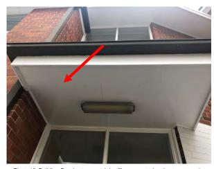
Photo 18: Building C, asbestos containing fibre cement sheeting to east and west entry soffits (R0013 & R0016)
