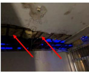
Photo 39: Building C, suspected SMF insulation throughout roof void
