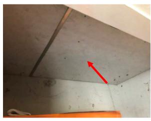
Photo 38: Building C, asbestos containing fibre cement sheeting to ceiling of Room R1004  $\,$
