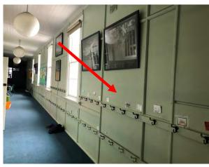
Photo 9: Building A, asbestos containing fibre cement sheeting go western wall of Room R1018
