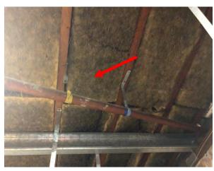
Photo 44: Building H, suspected SMF insulation to roof sarking
