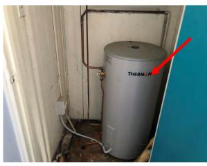
Photo 21: Building C, suspected SMF insulation core to hot water system in Room R0017
