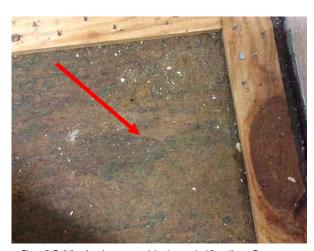
Photo 5: Building A, asbestos containing brown vinyl floor tiles to Room R1007
