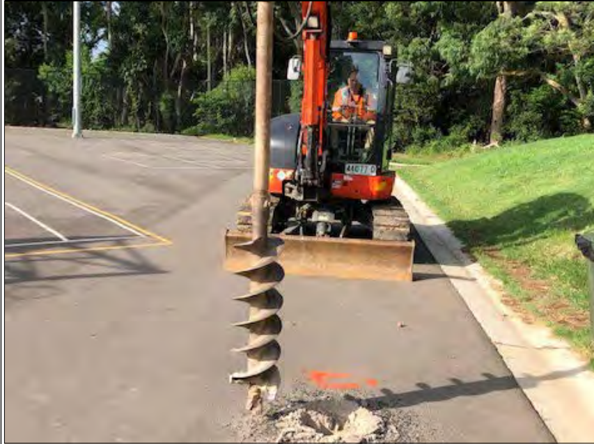
4. BH20 ISOLATED PATCHED HOLE WITH WARNING TAPE – 23.01.2019
