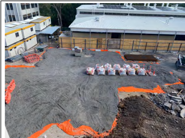
Photograph 1: Elevated view of marker layer installed beneath the High School Green.
