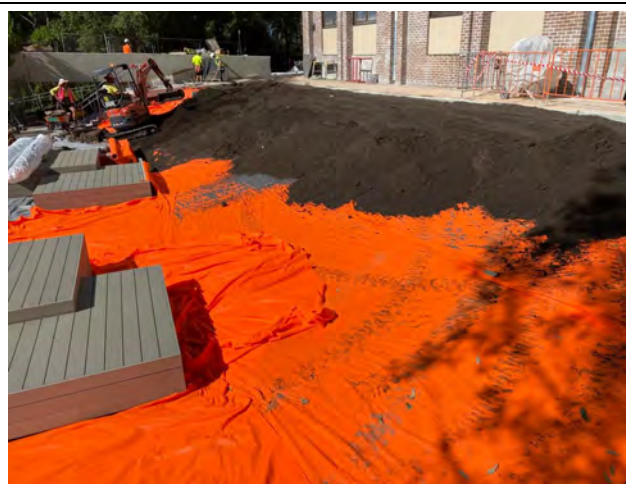
Photograph 2: Marker layer installed in landscaped area east of Building S.
