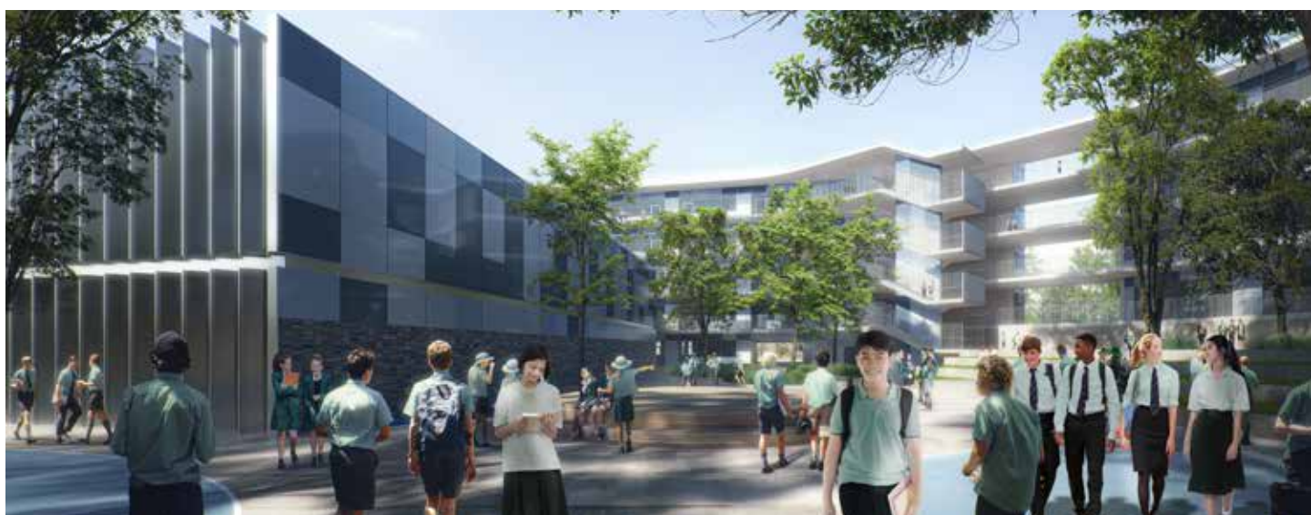
Artist impression of Cumberland High School buildings Z, Y, and X looking from the west.
