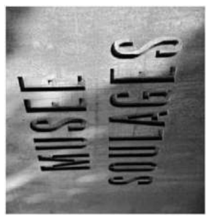
EXAMPLE OF CONCRETE SIGN WITH EMBOSSED LETTERING
