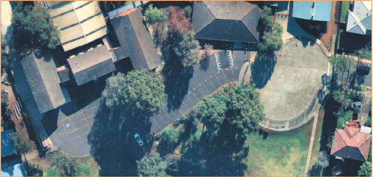
Figure 7: Existing CWPS Car Park (permanent condition) Source: Nearmap (dated 22 June 2018)
