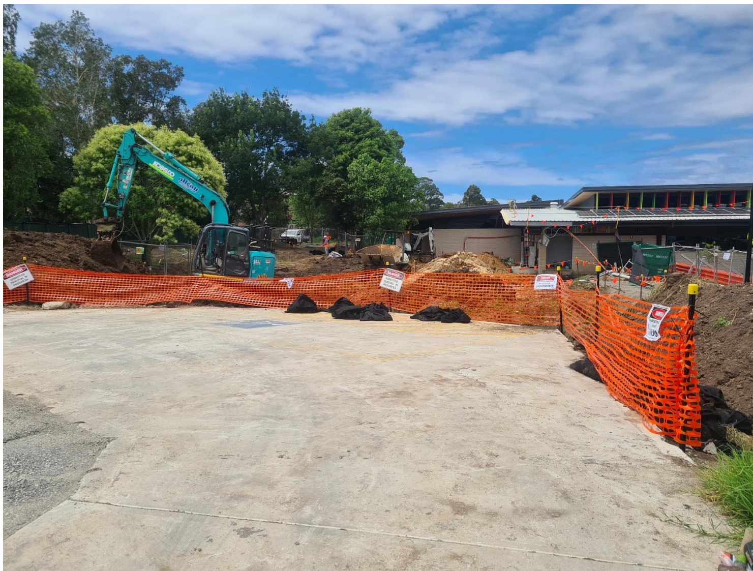
Figure 5: Asbestos removal area
