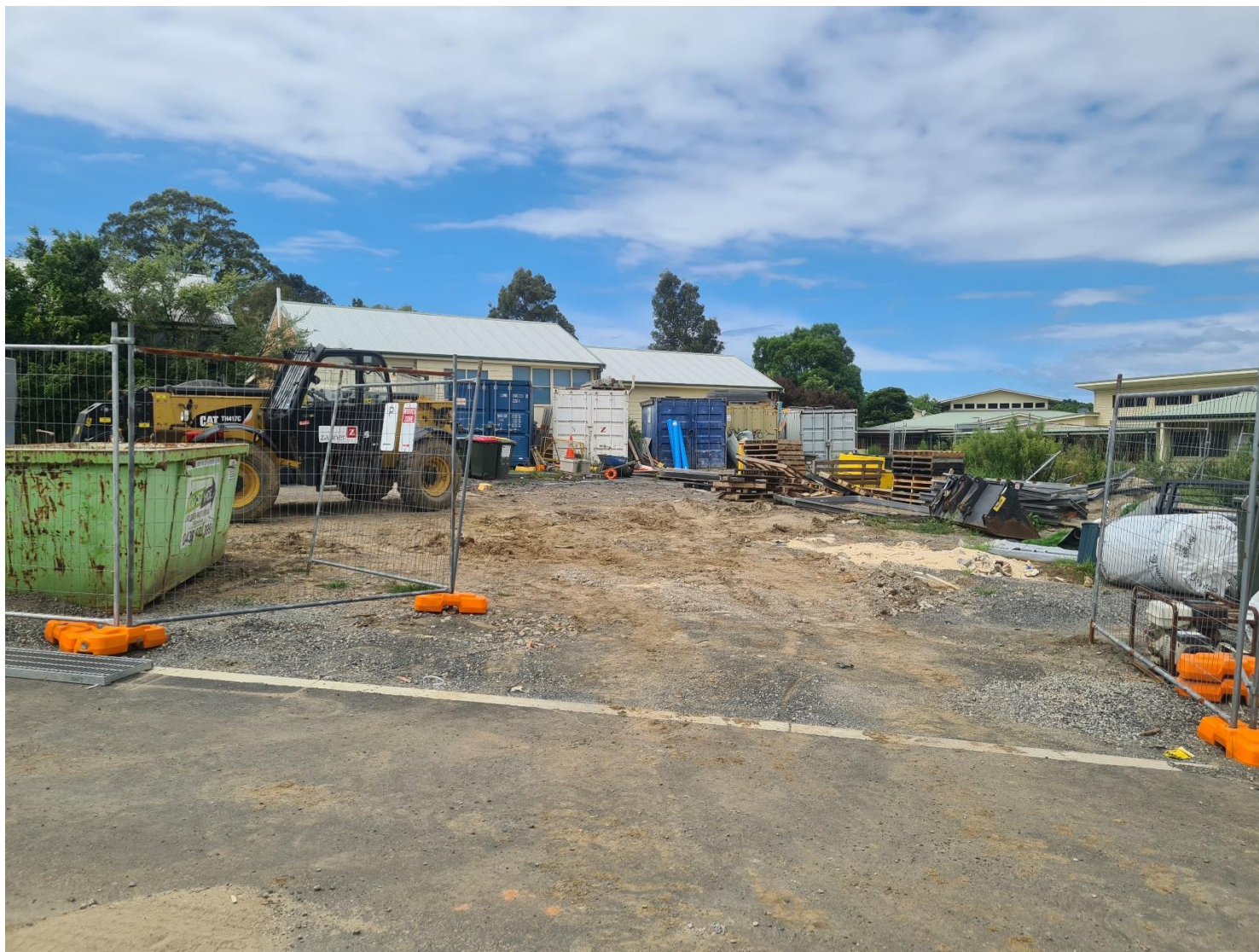
Figure 8: Waste storage area
