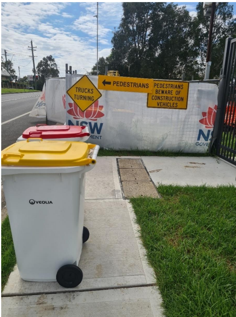
Figure 12: Hoarding in place
