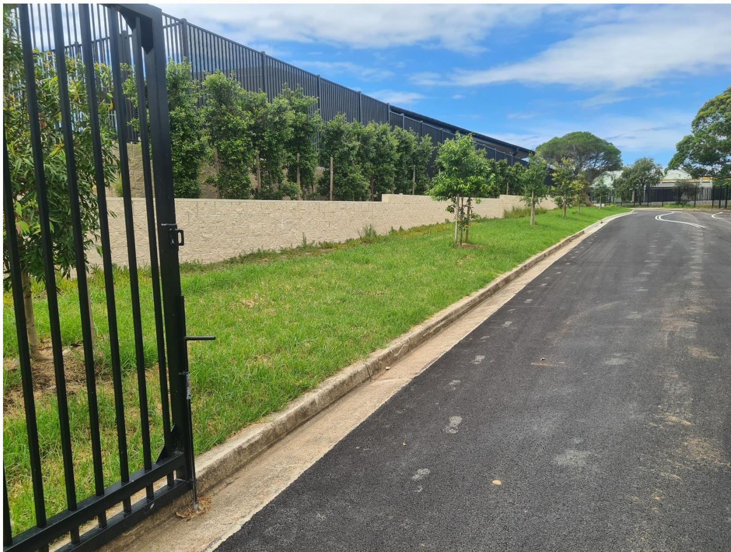
Figure 6: Previous erosion risk area, with landscaping complete
