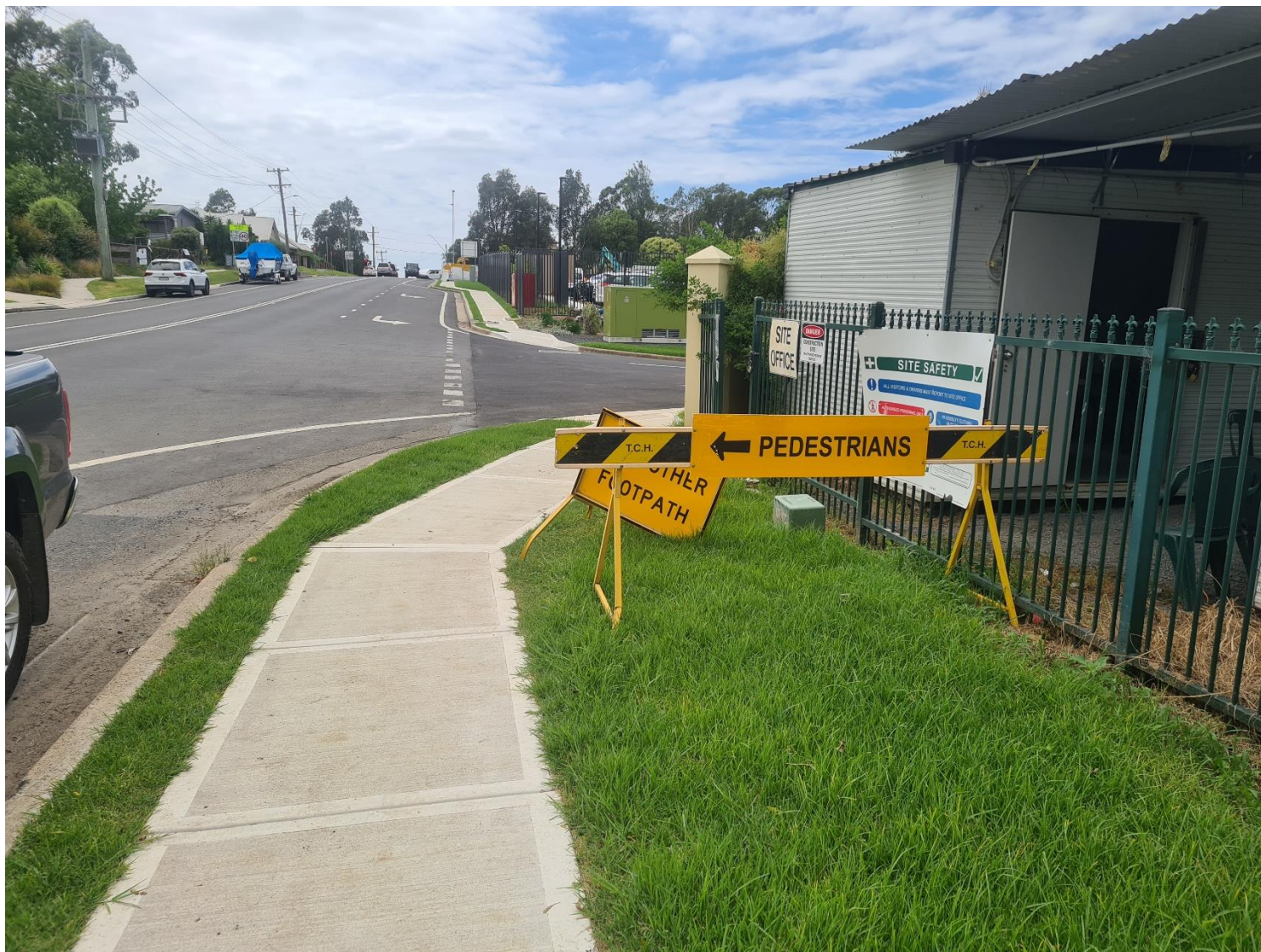
Figure 11: Footpath completed with turf alongside
