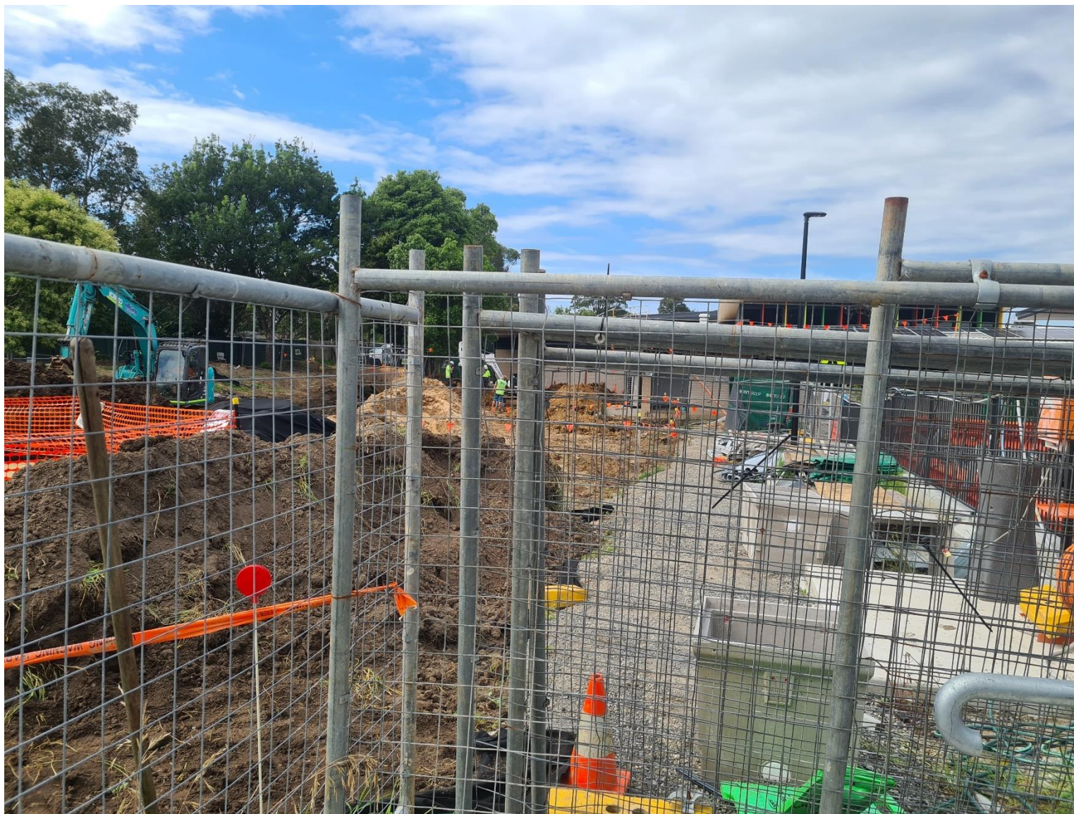
Figure 17: Hydrotherapy pool in construction
