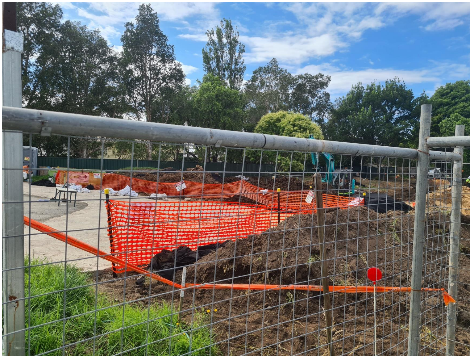
Figure 16: Hydrotherapy pool and construction area
