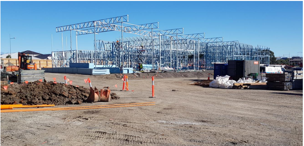
Photo 7: Hall structure being erected.
