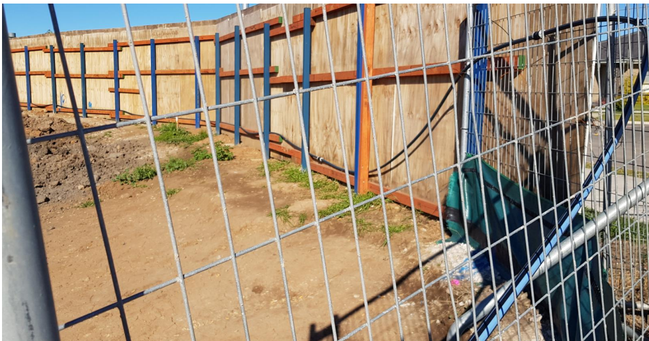
Photo 10: Black poly-pipe hose for dust suppression on permitter.
