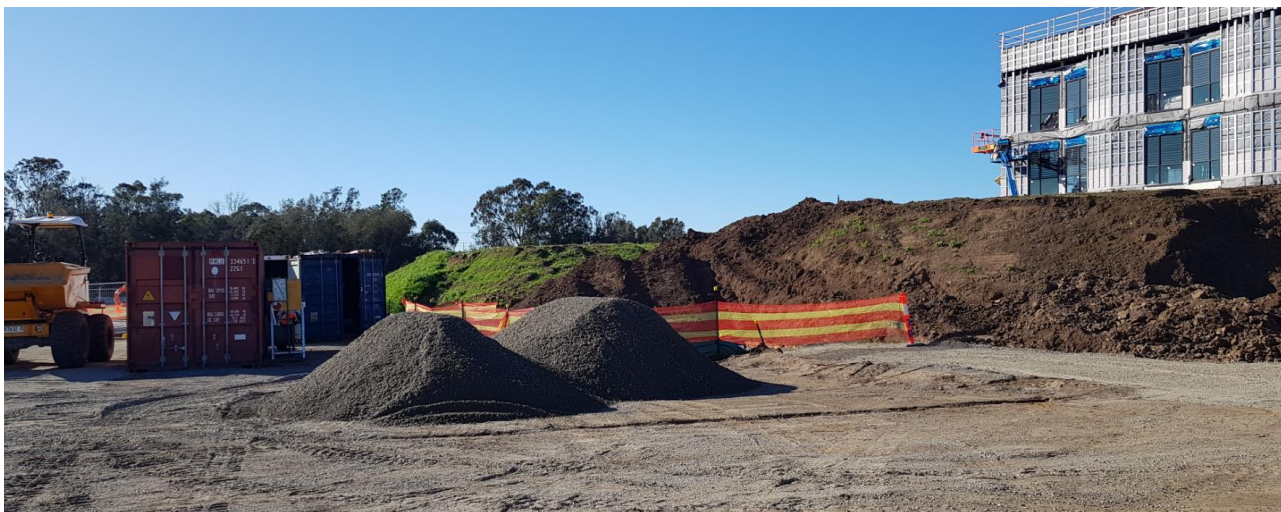
Photo 4: Material stockpiling. Note the stockpile stabilisation at rear (for static stockpile).
