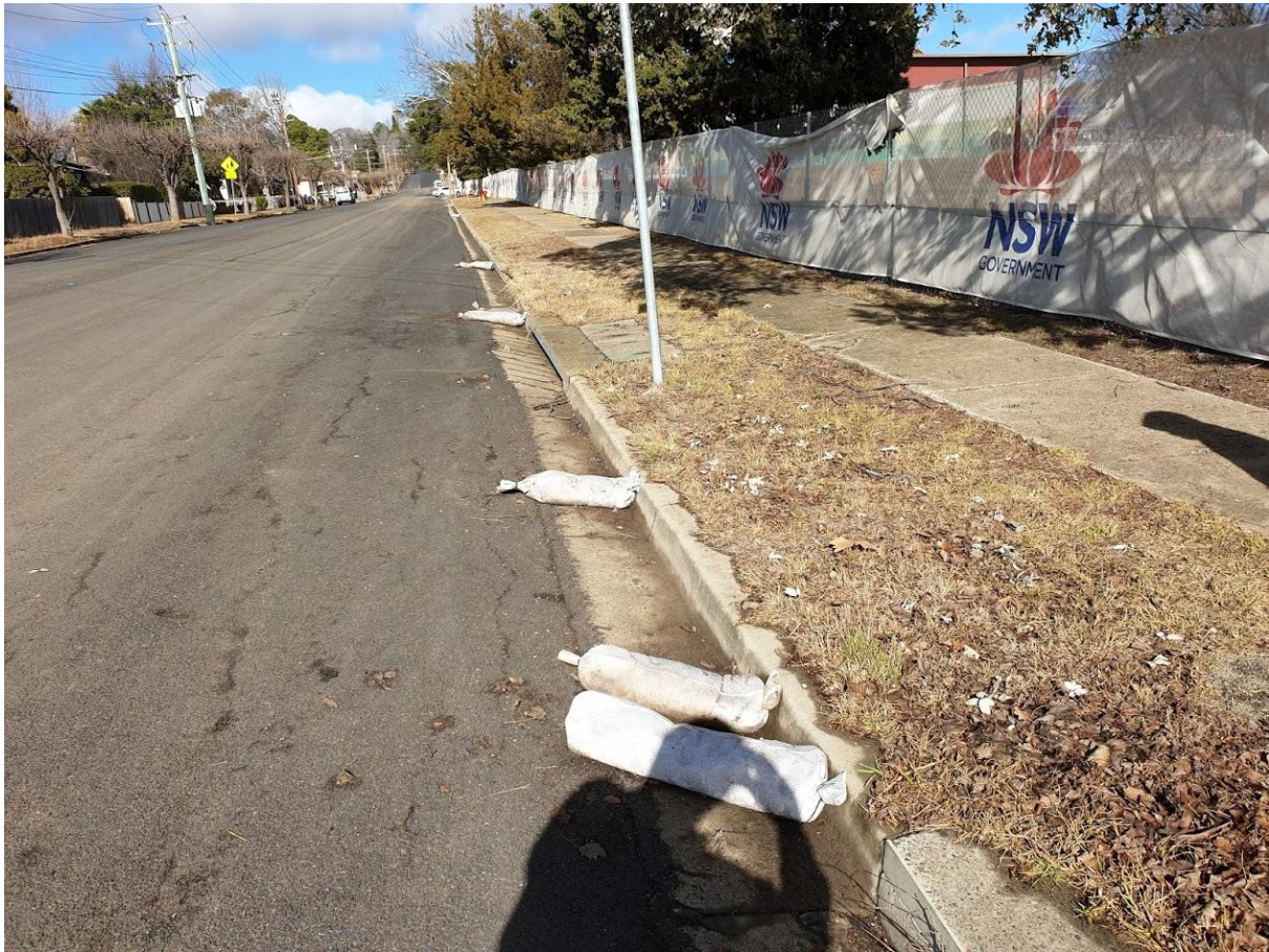
Plate 12 – Silt socks in Butler Street stormwater drain
