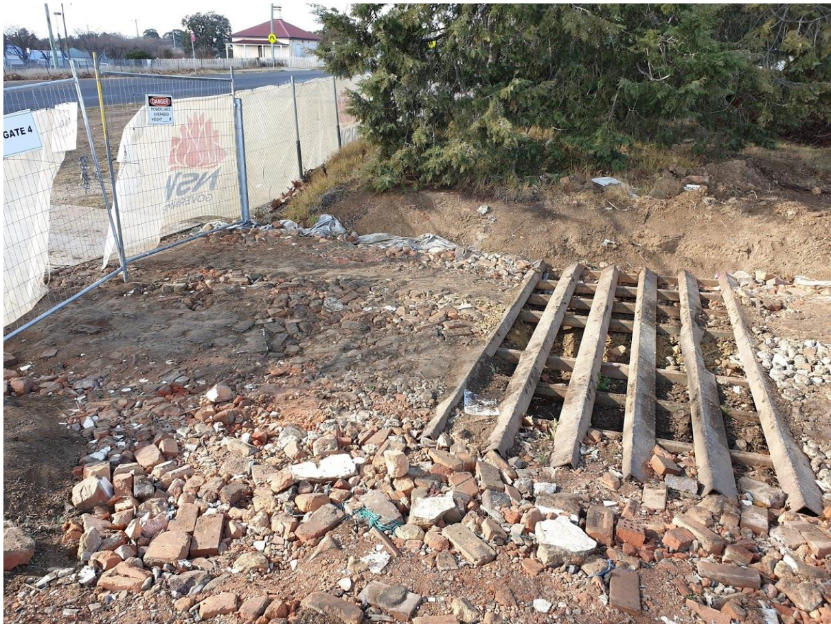
Plate 13 – Rumble grid and stabilized exit point at Gate 4
