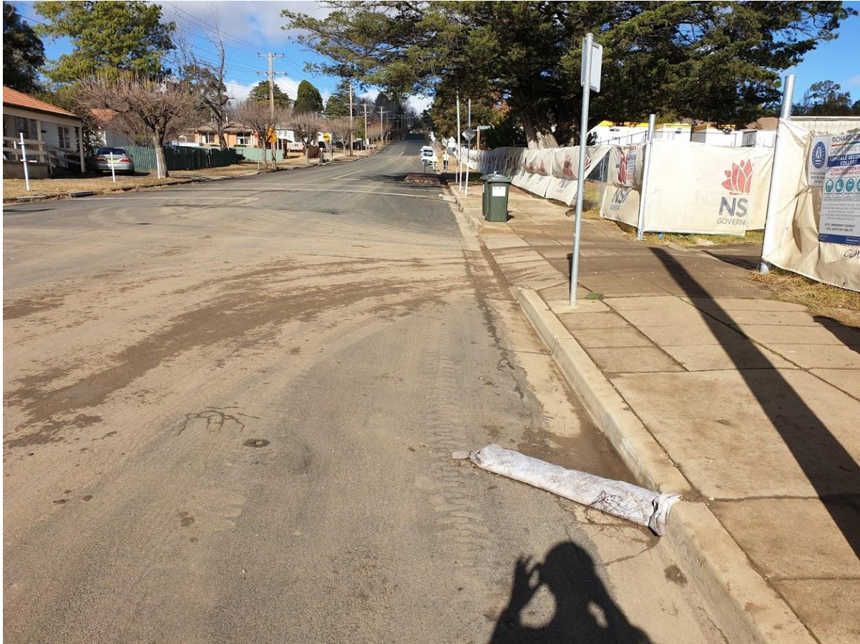
Plate 2 – Mud tracking from Gate 2 onto Butler Street
