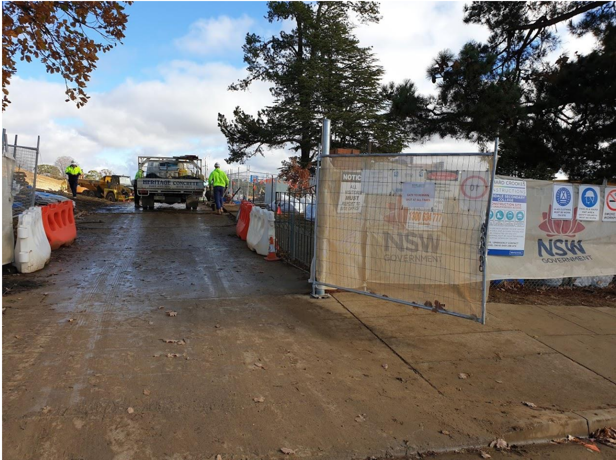
Plate 1 – Mud tracking over footpath onto Butler Street
