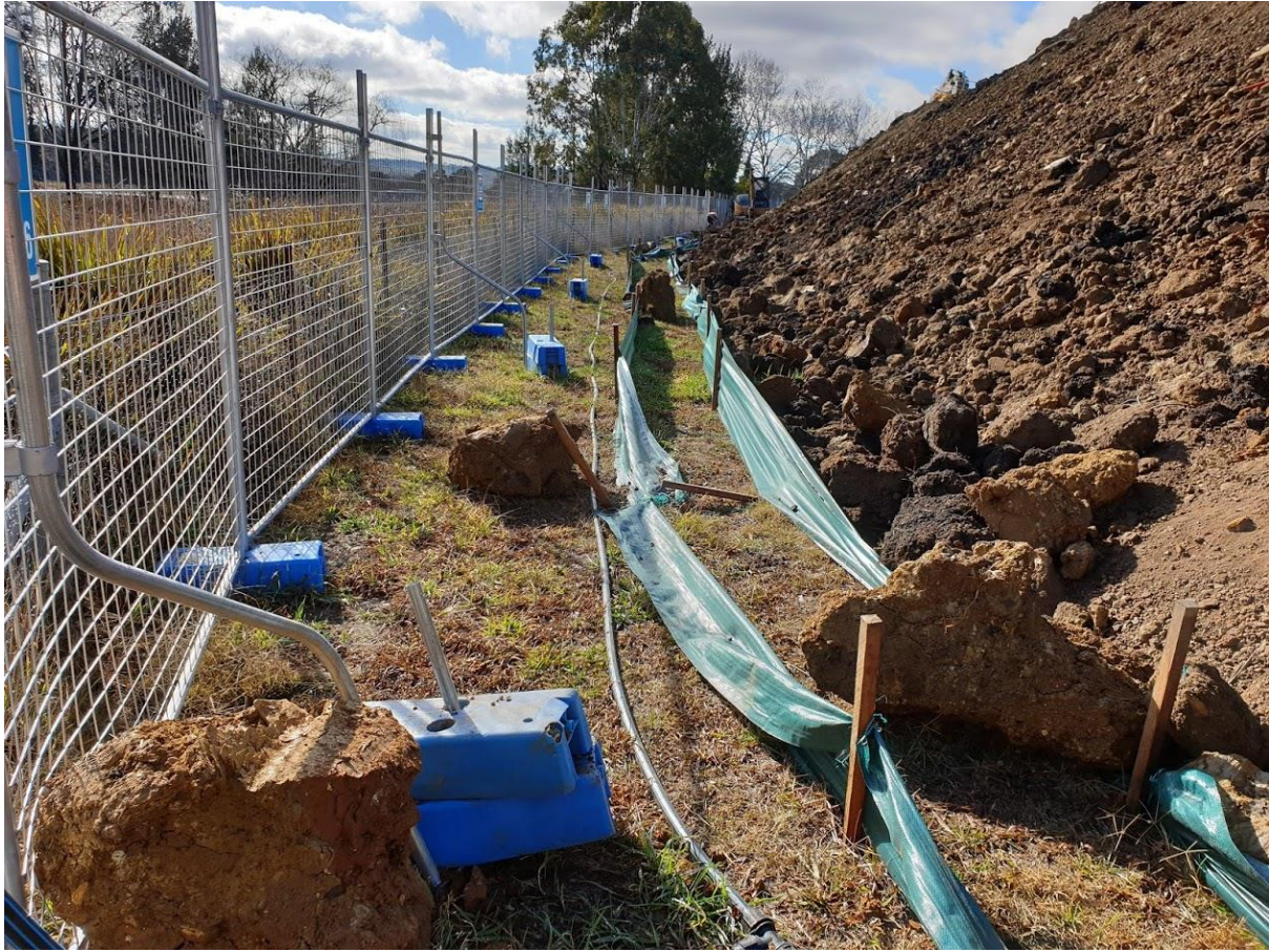
Plate 3 – Silt fence damaged by soil boulders
