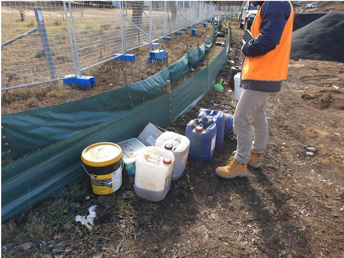
Plate 7 – Unknown chemical drums left in unbunded area
