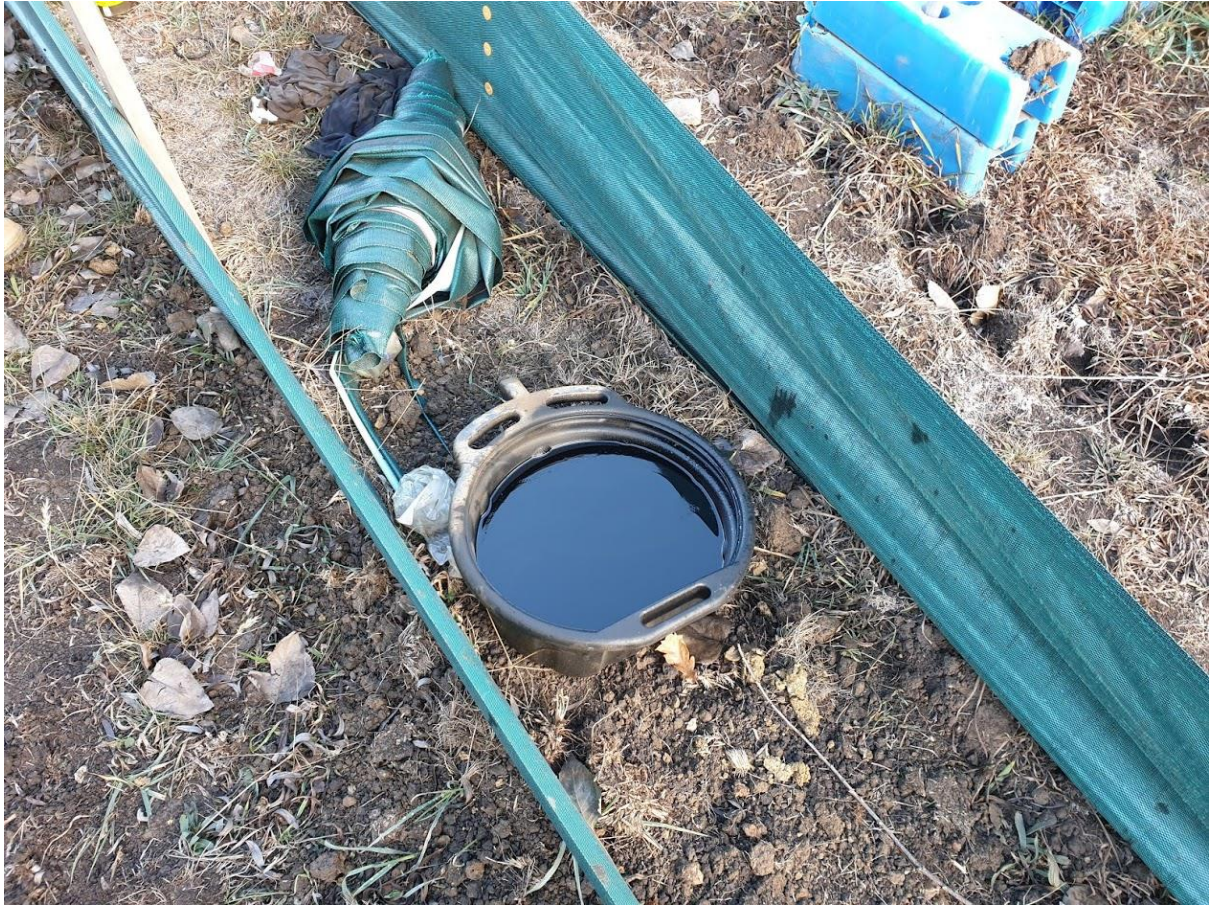
Plate 6 – Sump oil left in receptacle in non-bunded area
