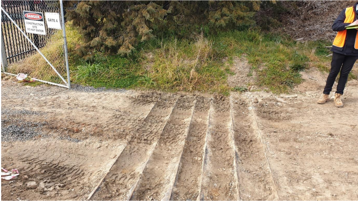
Plate 13 – Rumble grid at Gate 4 requires cleanout
