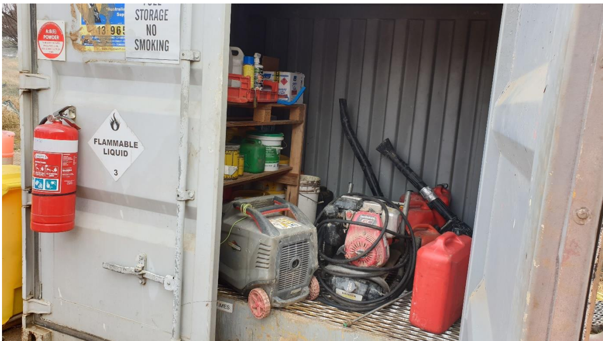
Plate 12 – Internally banded chemical store
