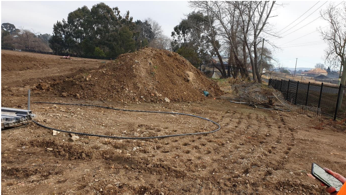
Plate 7 – Soil stockpile to north of oval without erosion and sediment controls on downslope side
