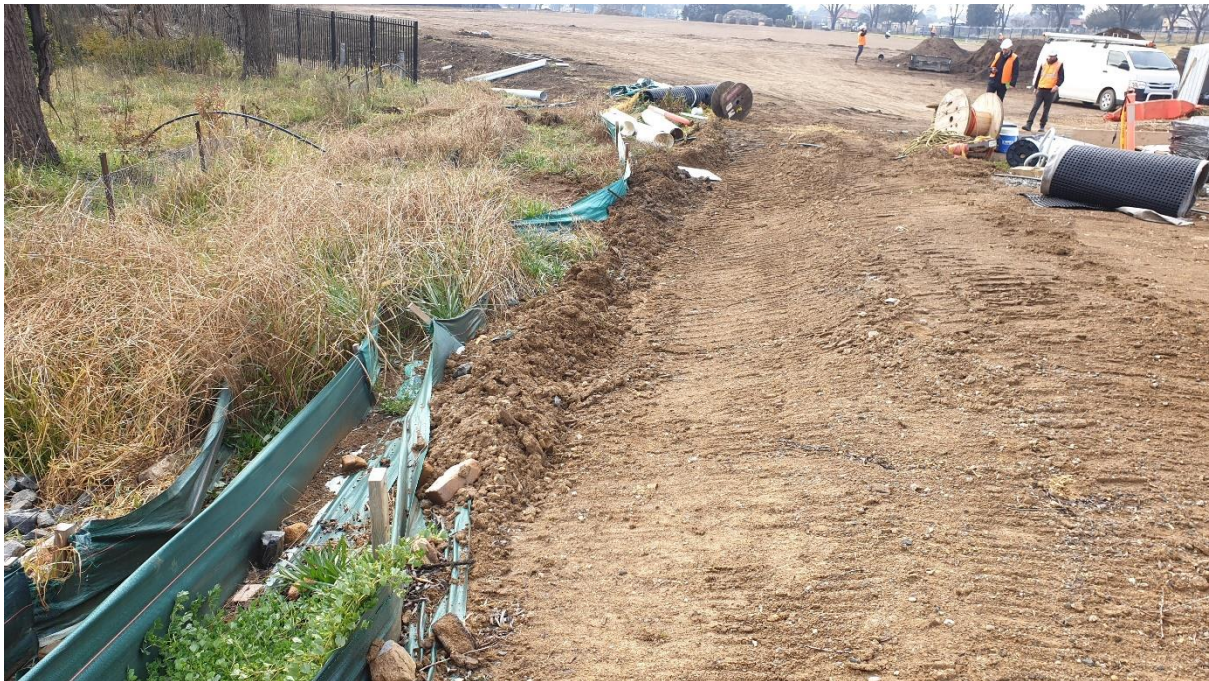
Plate 6 – Collapsed silt fence in drainage line leading to Wetland area
