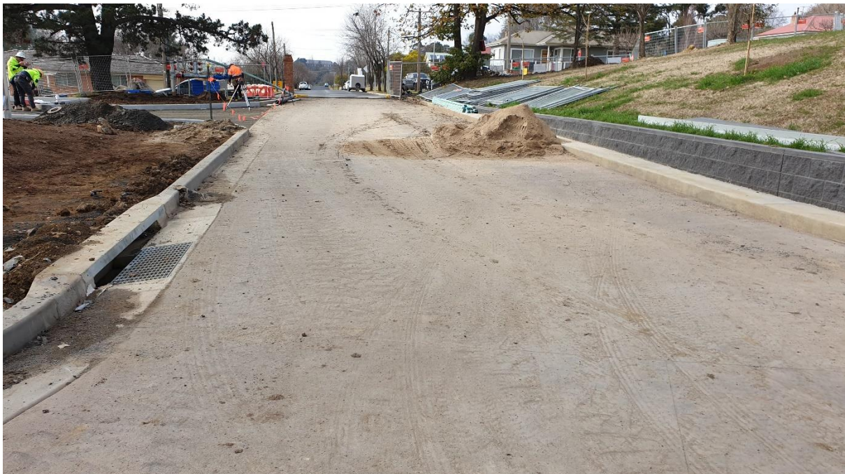
Plate 8 – Unprotected stormwater drain within active work area within the site
