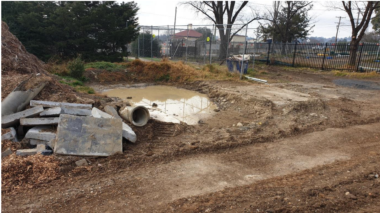
Plate 9 – Concrete washout pit
