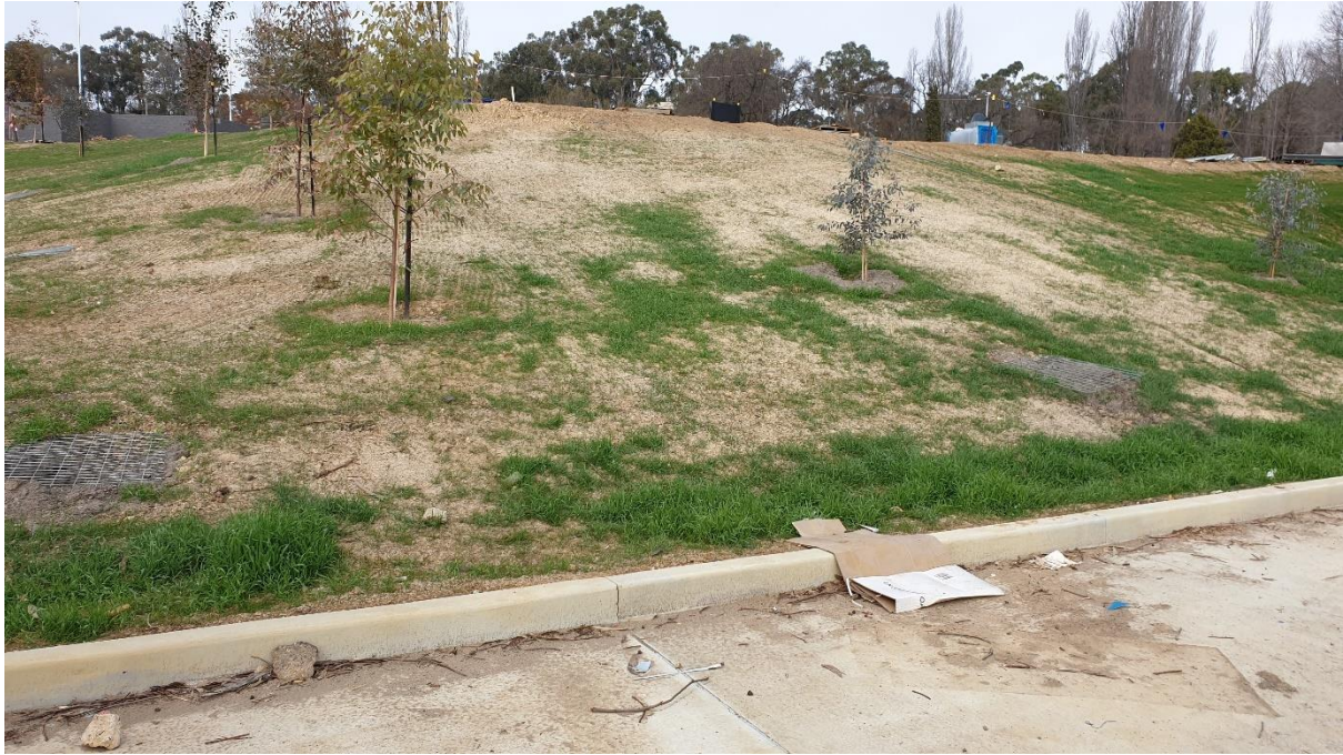
Plate 5 – Hydromulching stabilisation of batter slope
