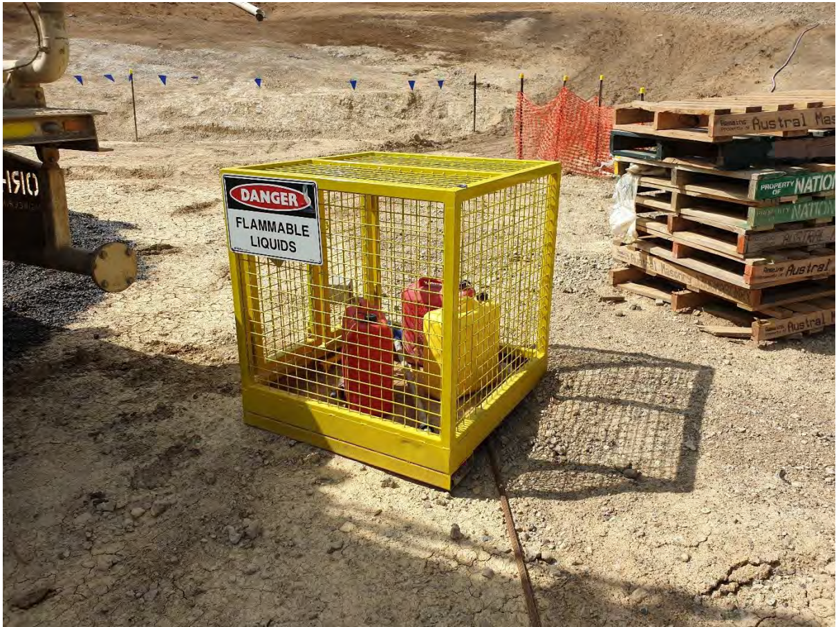
Plate 7 – Secure and bunded fuel storage cage
