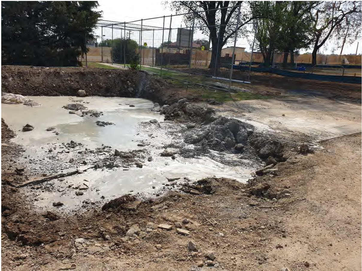
Plate 14 – Concrete washout pit
