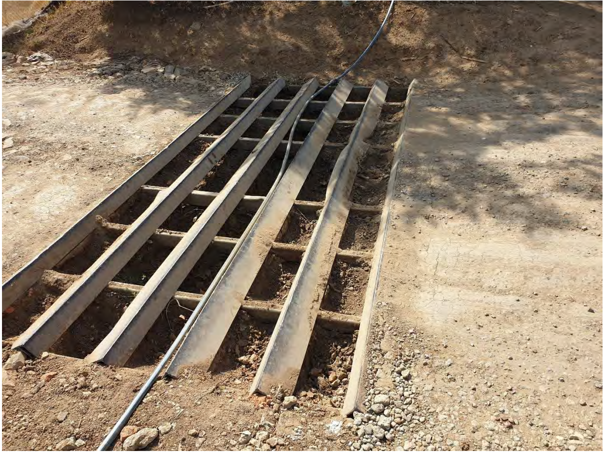
Plate 10 – Well maintained rumble grid
