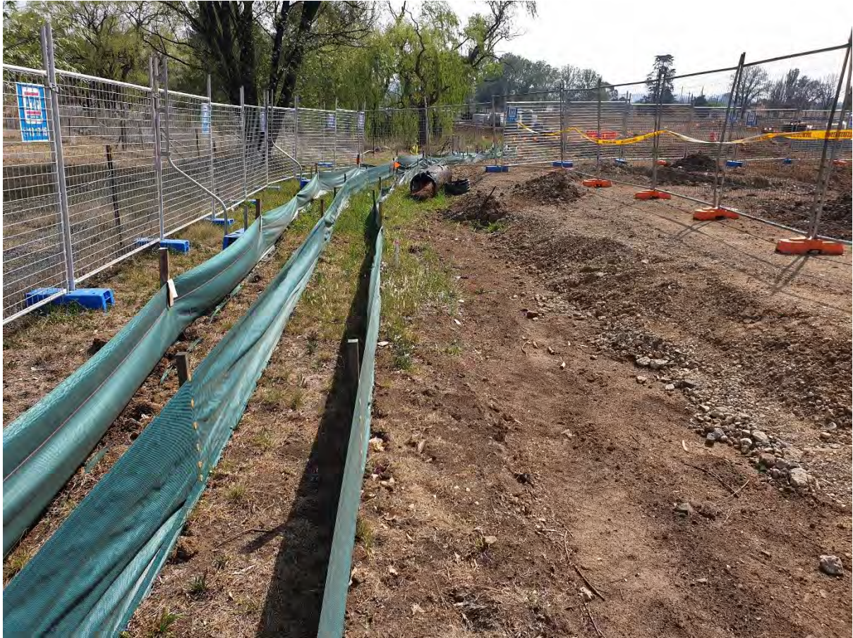
Plate 11 – Silt fencing
