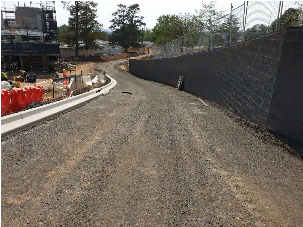
Plate 8 – Aggregate topped access road to reduce dust emissions
