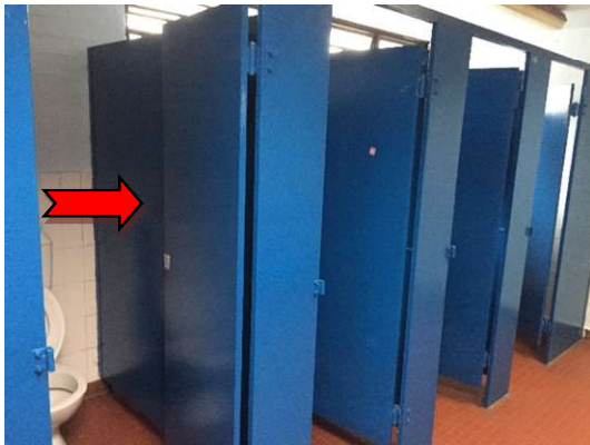
Photograph 7: Asbestos containing fibre cement.
