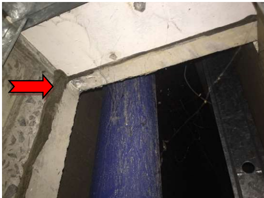
Photograph 3: Asbestos containing construction joint mastic.
