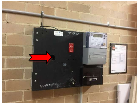
Photograph 4: Asbestos containing fibre cement sheeting.
