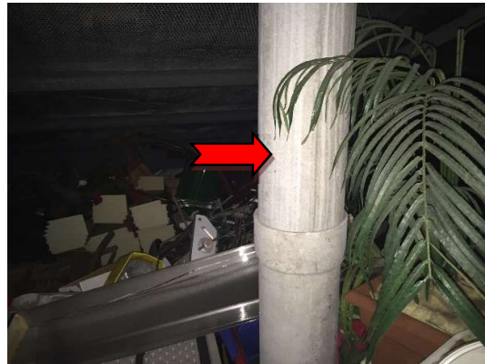
Photograph 8: Asbestos containing moulded fibre cement.
