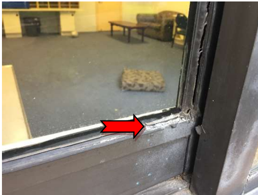
Photograph 3: Asbestos containing construction joint mastic.
