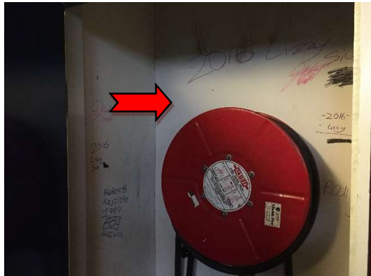
Photograph 4: Asbestos containing fibre cement sheeting.
