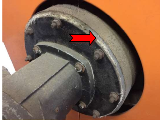
Photograph 8: Asbestos containing moulded fibre cement.
