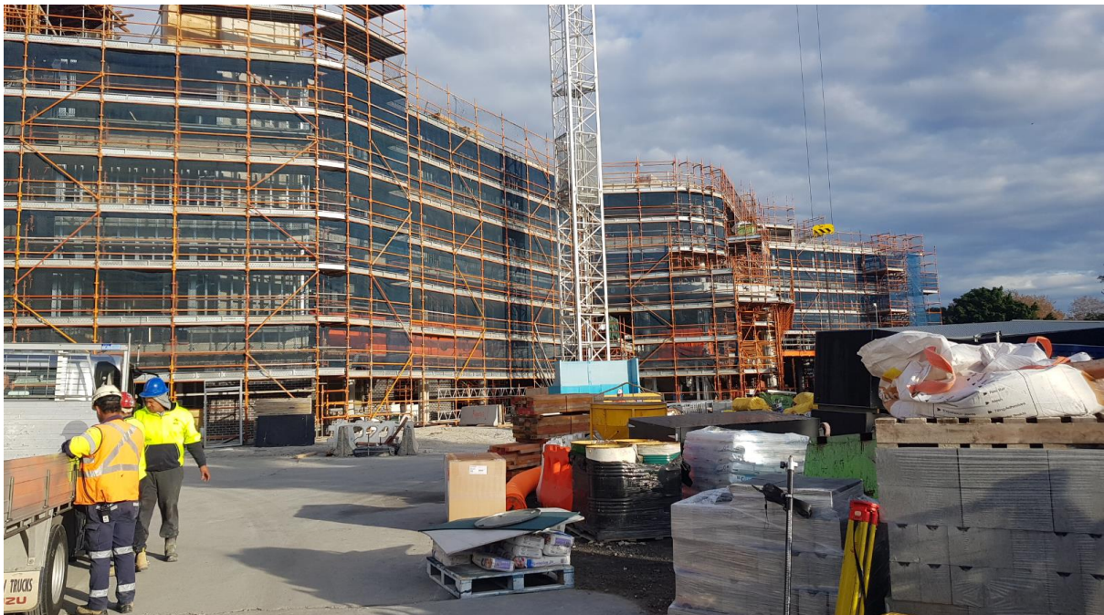
Photo 2: Phase 1 structure erected to level 3. Fit-out underway.
