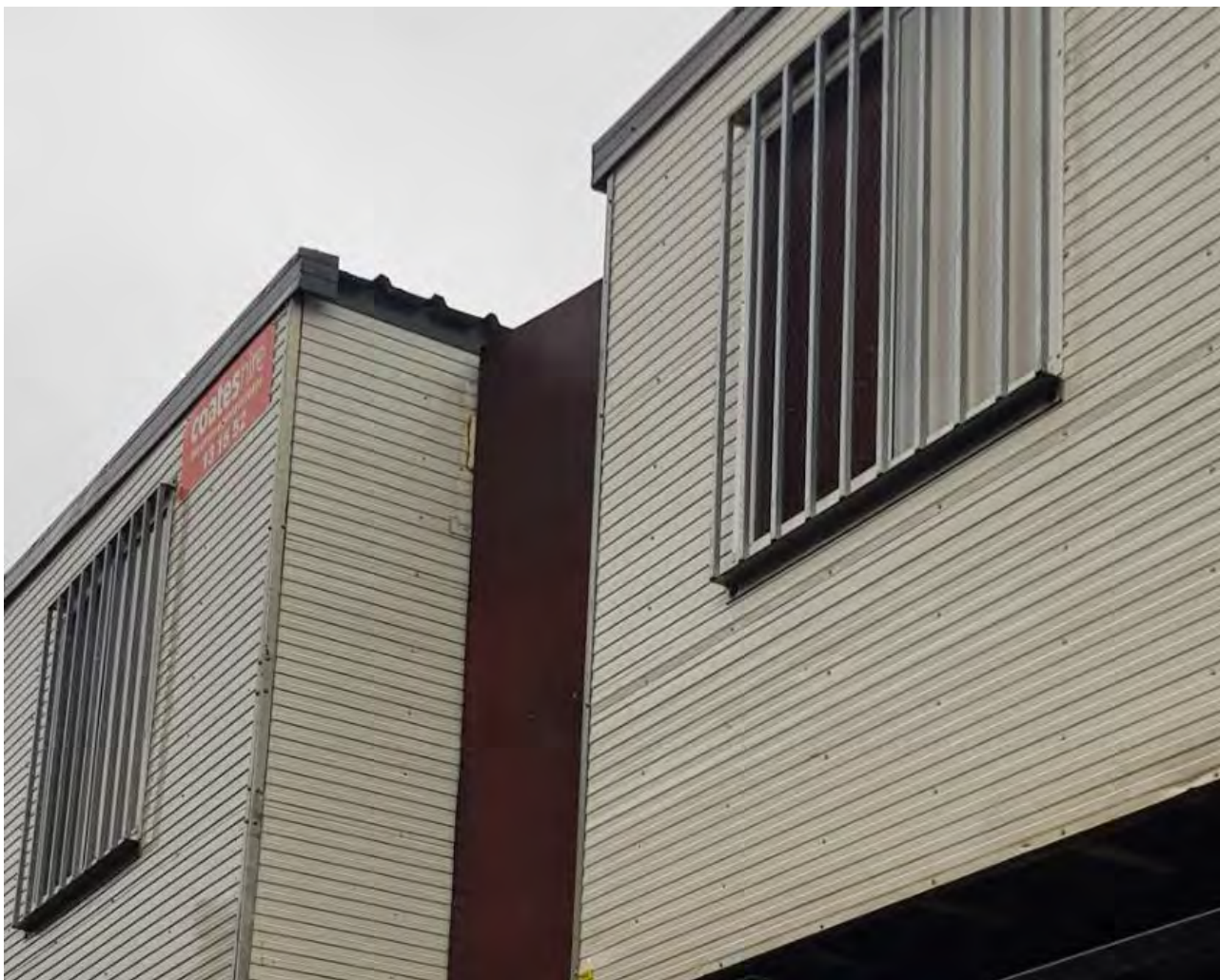
Photo 4: Site hut windows boarded for privacy and hoarding between huts for noise attenuation.
