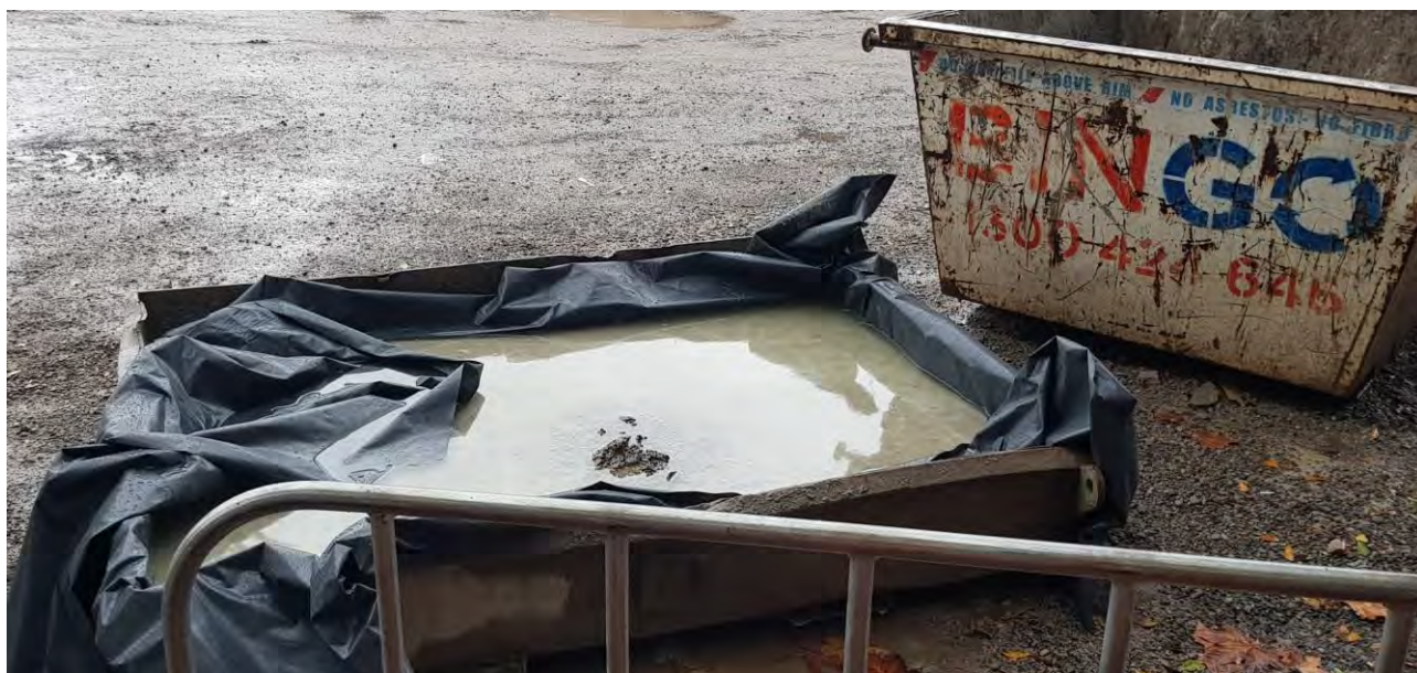
Photo 3: Concrete washout tray.
