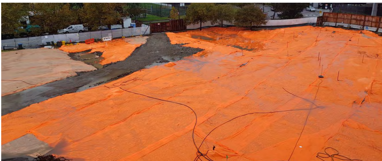
Photo 5: Geofabric on asbestos impacted soils. Rock on haul road and sprinklers erected.
