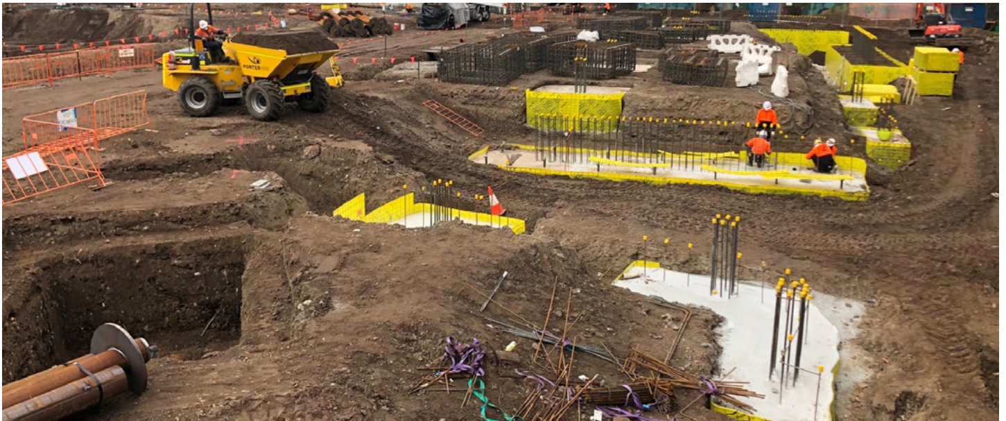
Installation of groundfloor pilecaps and concrete pouring
