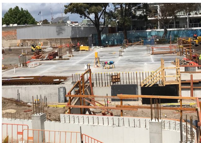
The first concrete capping slab has been poured
