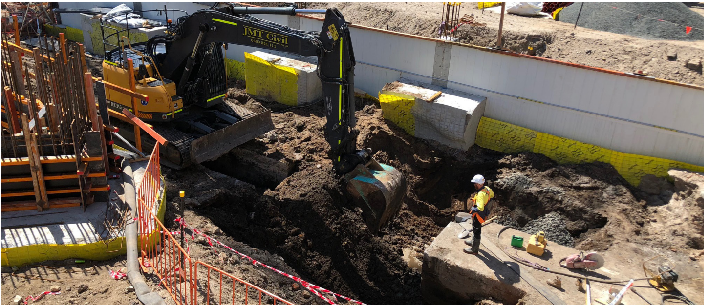
Works commenced to the stormwater culvert passing through the site
