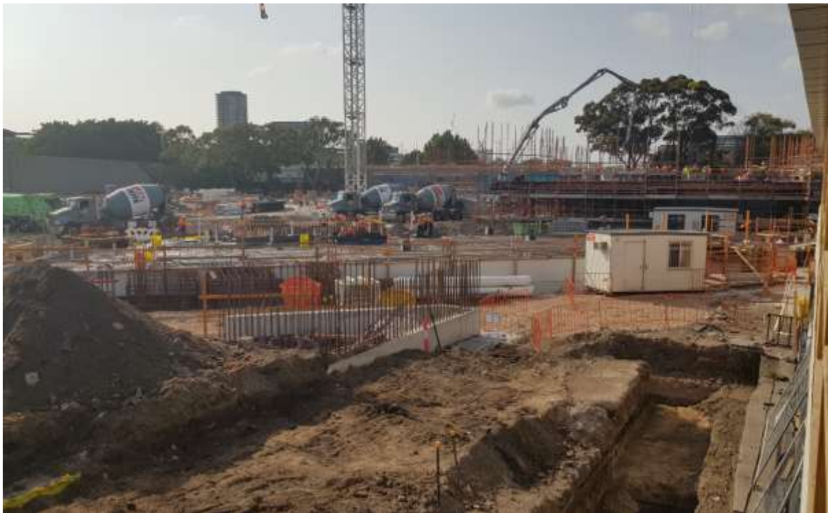
Photo 3: First floor pour, with tower crane erected.
