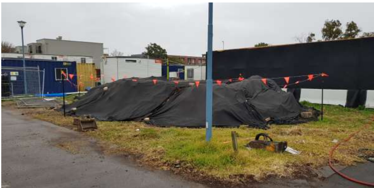
Photo 12: GSW stockpile stabilization
