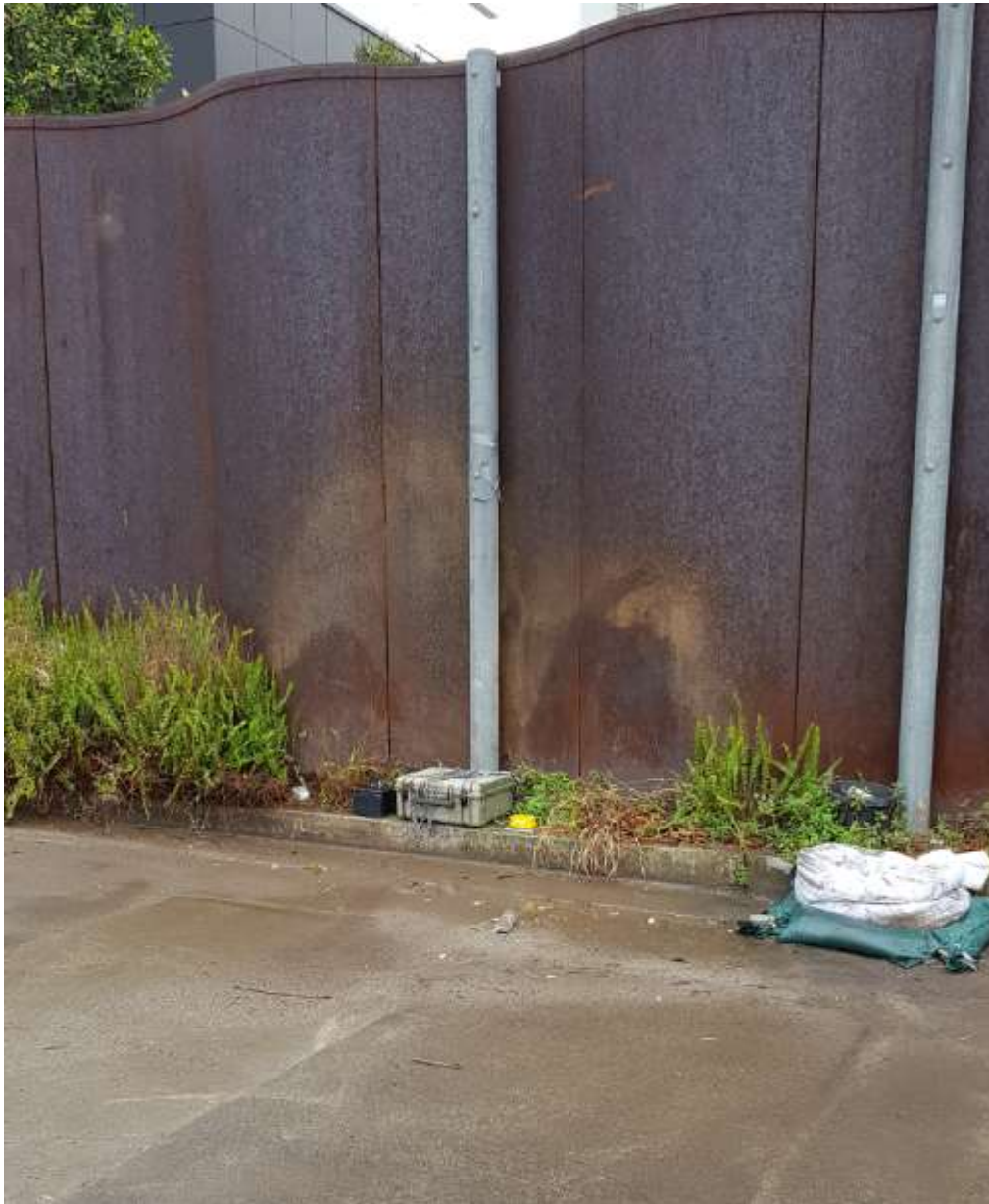
Photo 8: Vibration monitoring and drain protection
