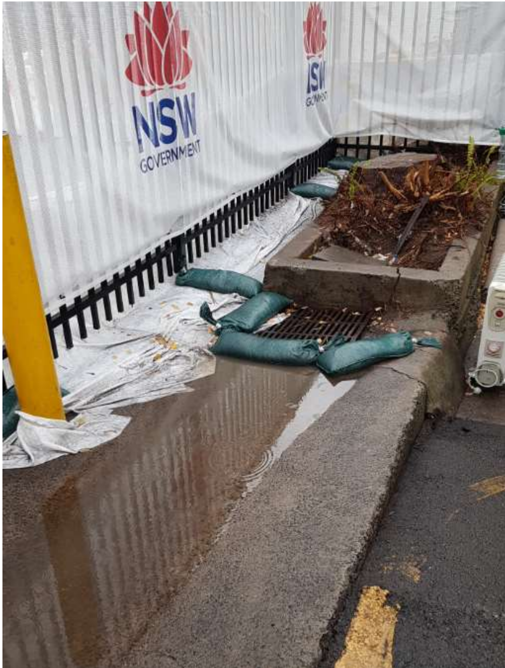
Photo 2: Erosion and sediment control
