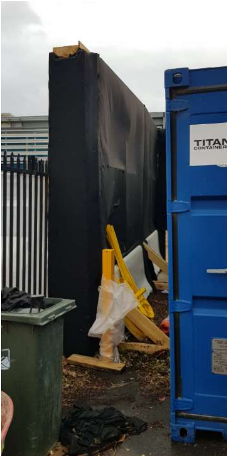
Photo 4: Noise barrier on boundary with existing school.
