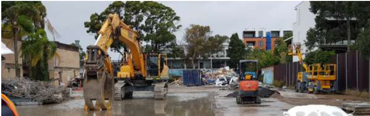
Photo 5: Material segregation. Note proximity of works to receivers on western (right of shot) and southern (centre) boundaries
