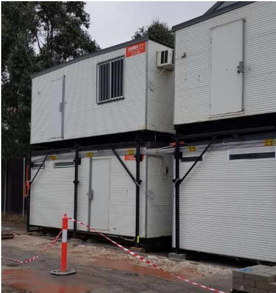
Photo 6: Site sheds are being installed to provide extra privacy and noise attenuation for properties on western boundary
