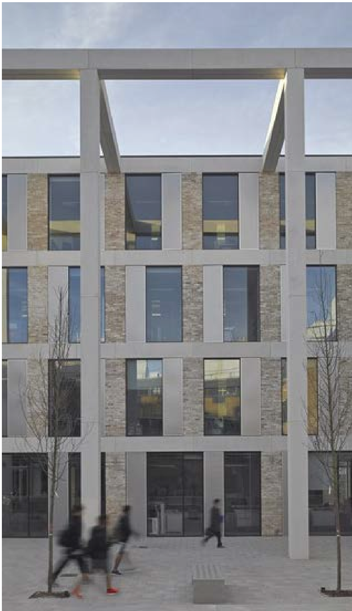
Concrete framed structure
