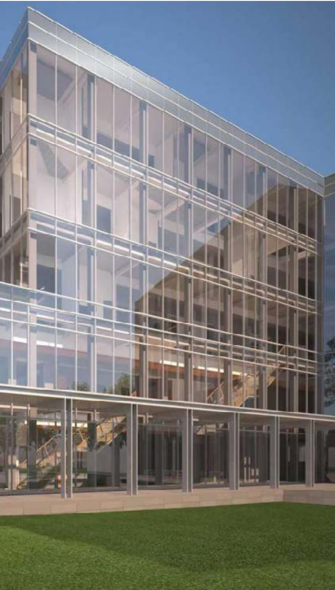
Steel framed structure
