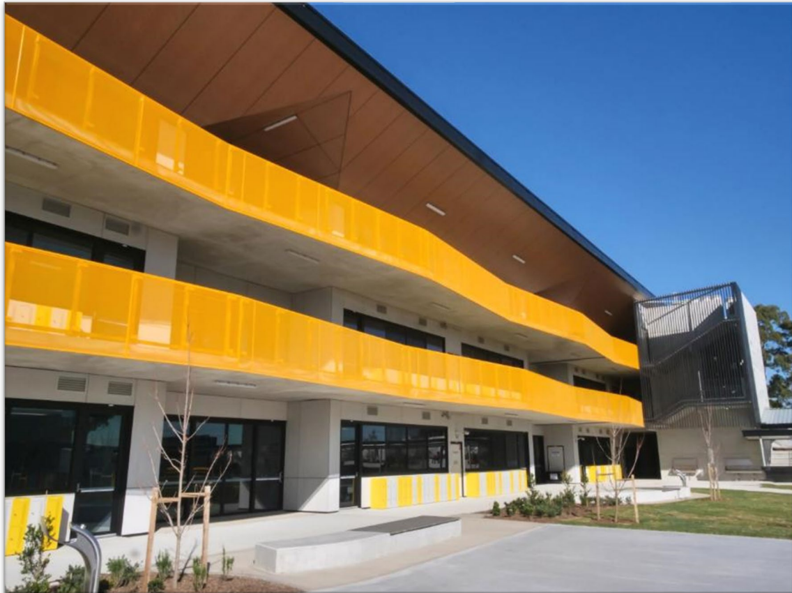
Figure 16: The new 3-storey building at Canterbury South Public School opened for students and teachers in 2021.
