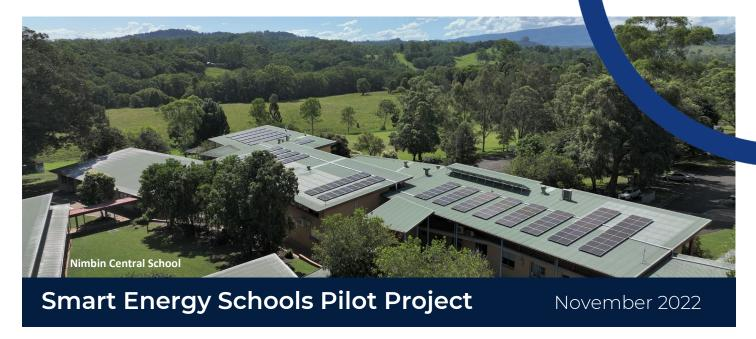
Solar and battery energy storage systems and air conditioning units with smart controls have now been installed at 24 schools taking part in the first stage of the Smart Energy Schools Pilot project.
