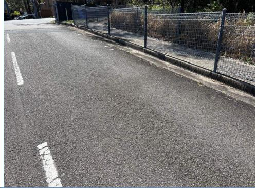
General views of the kerb, gutter and road surface showing crack damage throughout.
