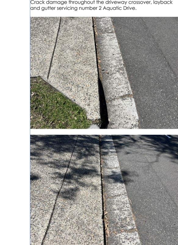
Crack damage throughout the driveway crossover, layback
