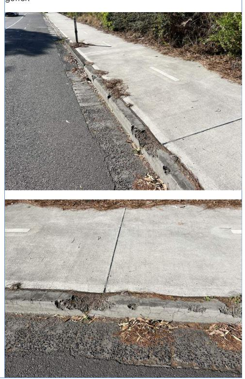
90m Various sections of crack damage throughout the kerb and gutter.
