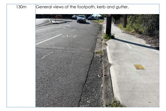
Crack damage throughout the kerb and gutter.
