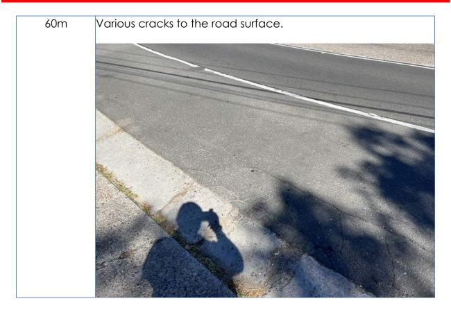
60m Layback and gutter showing multiple cracks.
