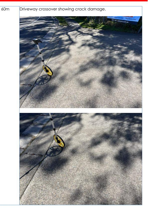
60m Driveway crossover showing crack damage.
