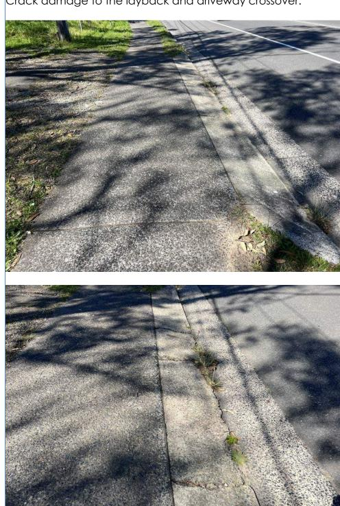
25m Crack damage to the layback and driveway crossover.
