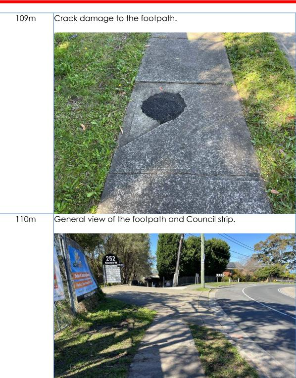
Crack damage to the footpath.
