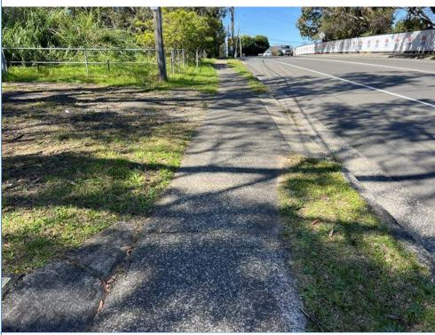
23m Crack damage to the footpath.
