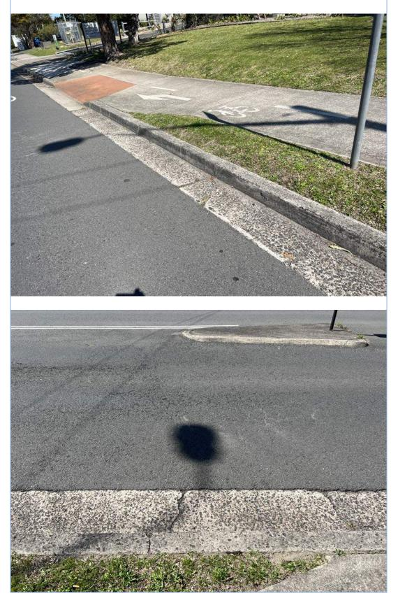
Crack damage noted to the kerb and gutter between the bus stop and the driveway servicing number 187 Allambie Road, Allambie Heights.
