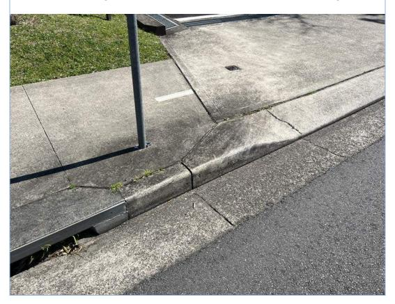
Crack damage throughout the road surface to the south of the driveway servicing number 187 Allambie Road, Allambie Heights. Crack damage throughout the road surface to the south of the driveway servicing number 187 Allambie Road, Allambie Heights. Views of the footpath between the driveway servicing number 187 Allambie Road and the bus stop to the western side of Allambie Road, Allambie Heights.
