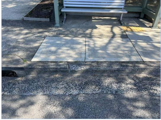
Crack damage to the footpath, kerb and gutter fronting the bus stop.
