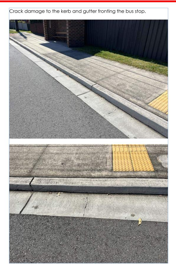
Crack damage to the kerb and gutter fronting the bus stop.
