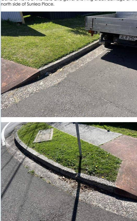
General views of the kerb and gutter showing crack damage at the
