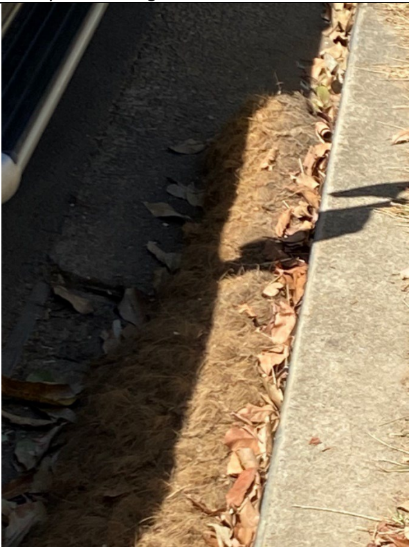
Photo 3: Coir sediment protection on the drain along Glenwood Park Drive (adjacent to site)
