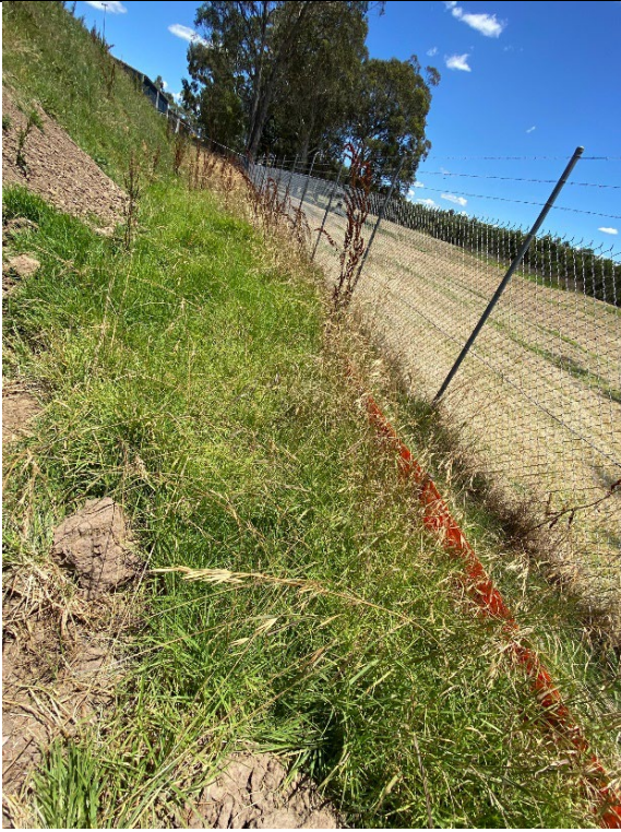
Photo 7: Sediment fence along the northern boundary of the topsoil stockpile
