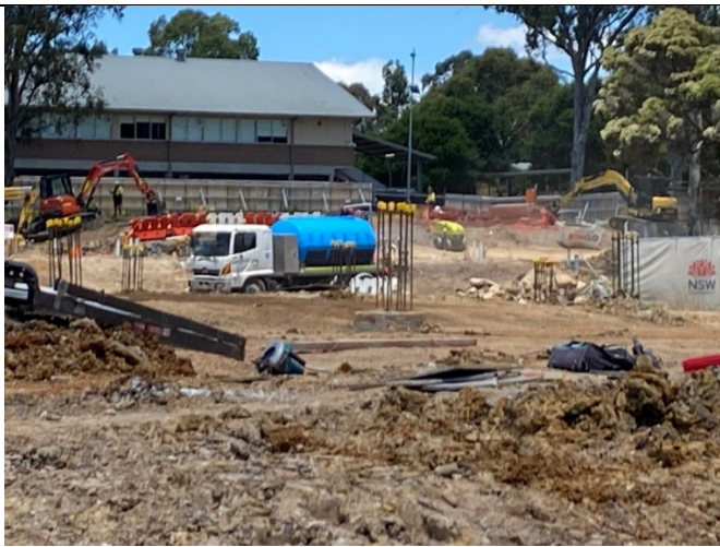
Photo 27: Water tanker for dust management
