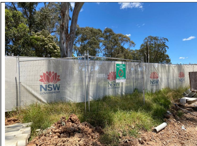
Photo 11: Boundary fence along Vegetation Zone 1 (fence extension to provide a 5m TPZ from the tree located inside the fence)
