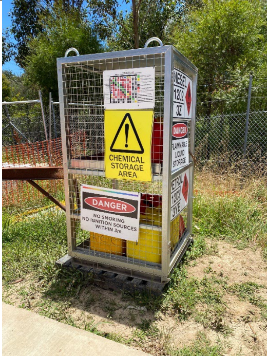
Photo 30: Chemical storage cage (bundled and locked)
