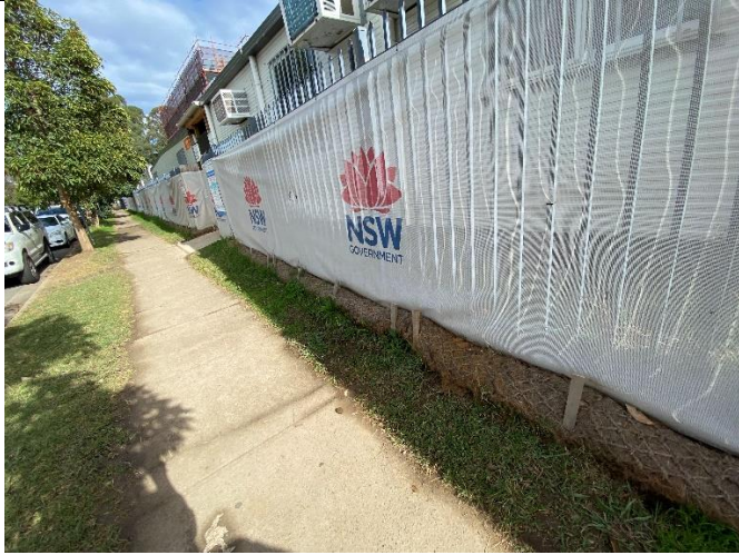
Photo 1: Coir sediment protection outside the boundary fence along Glenwood Park Drive
