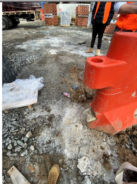
Photo 29: Concrete pad made with excess concrete to stabilise the truck turning area in the north east of the site (A2_NC05)
