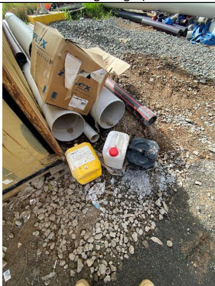
Photo 27: Chemicals located outside of bunding and without labelling (A2_IO3)
