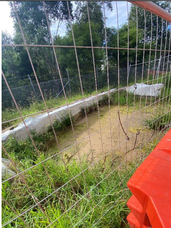
Photo 3: Basin with wash-off water from the rumble grid at the site entrance (A2_IO6)
