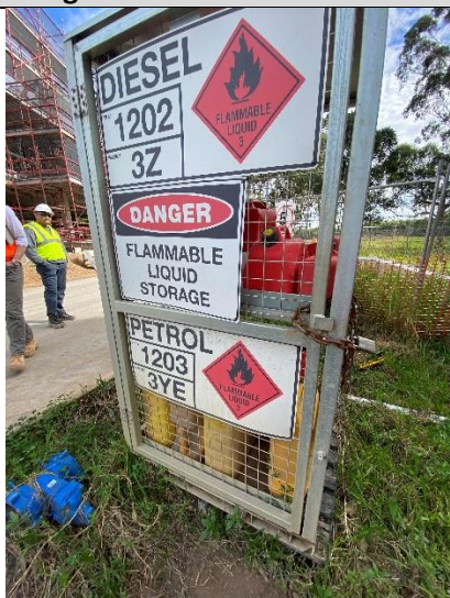
Photo 25: Chemical storage cage (bunded and locked)
