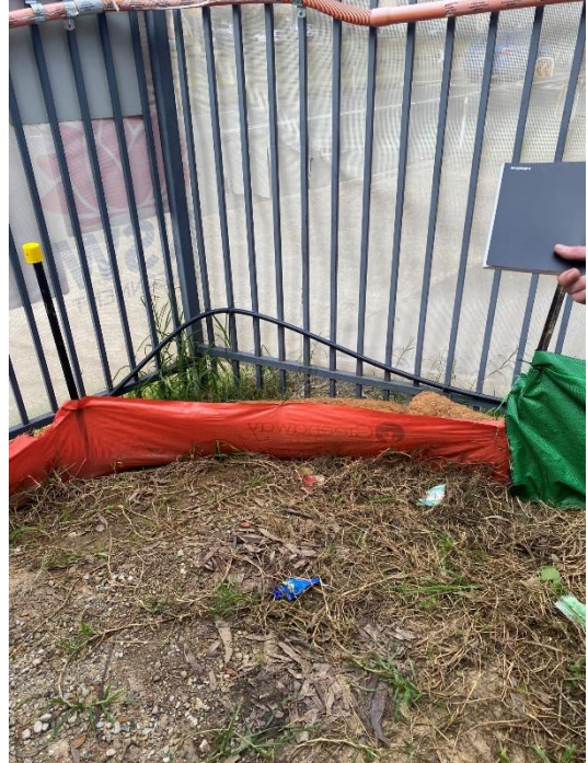
Photo 6: Sediment fencing along the eastern site boundary, south of the site office
