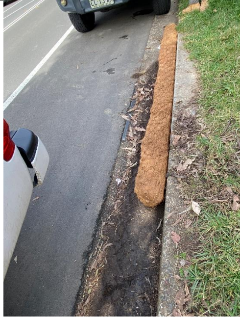
Photo 2: Coir sediment protection on the drain along Glenwood Park Drive (adjacent to site)
