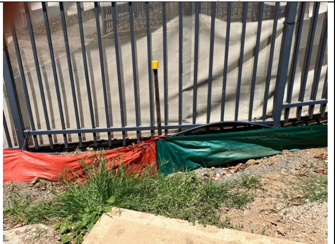
Photo 41: Evidence of sediment fence repairs
