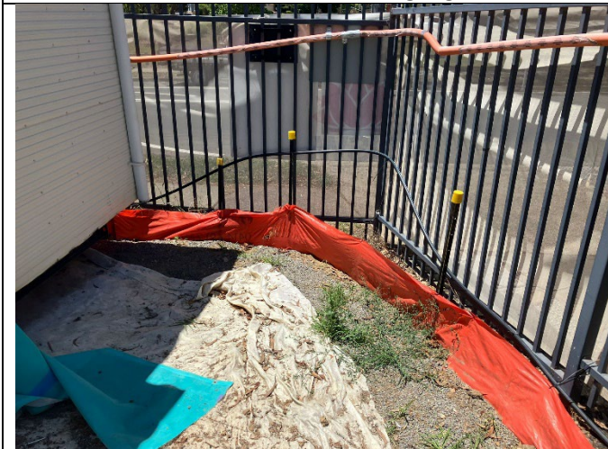
Photo 40: Evidence of sediment fence repairs
