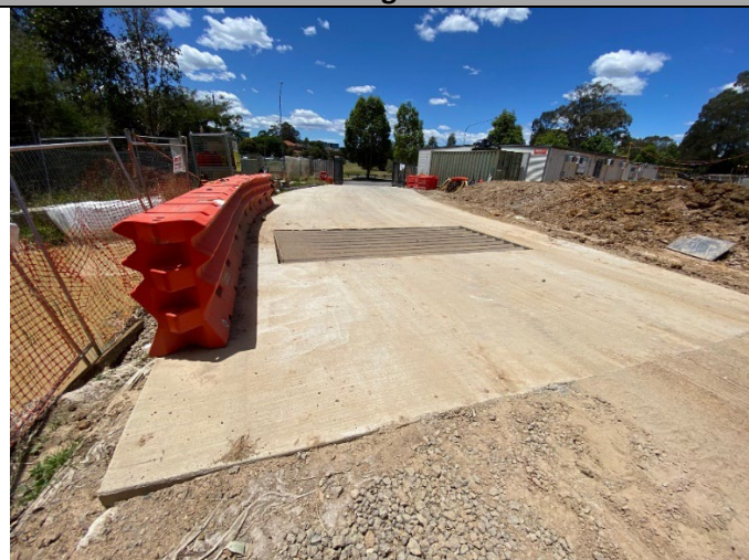
Photo 23: site entrance rumble grid and wheel wash (water drains to a small holding pond behind the fencing)
