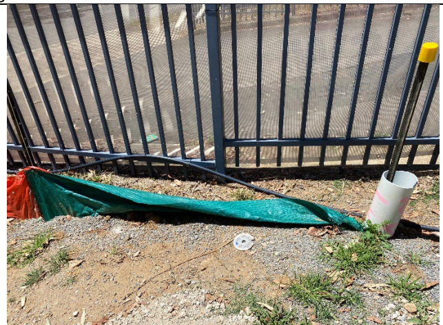
Photo 6: Sediment fencing along the eastern site boundary, south of the site office (noting poor condition)
