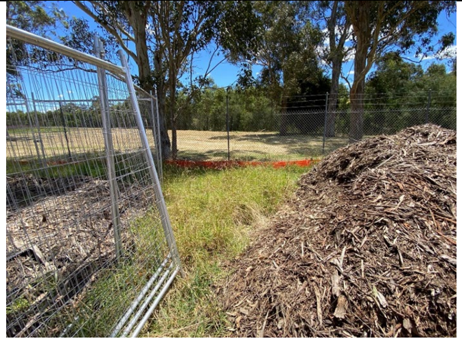
Photo 8: Sediment fence along the northern boundary of the site
