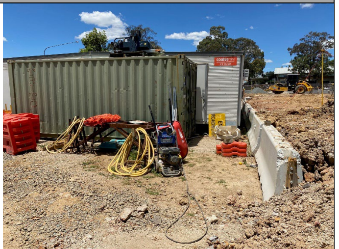
Photo 24: Hose and pump for the wheel wash, adjacent to the rumble grid
