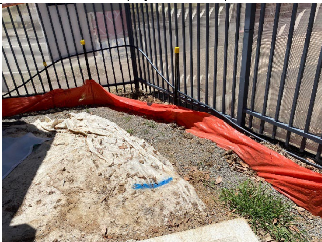
Photo 5: Sediment fencing along the eastern site boundary (south of the site office)
