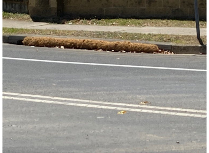
Photo 2: Coir sediment protection on the drain along Glenwood Park Drive (opposite the site entrance)
